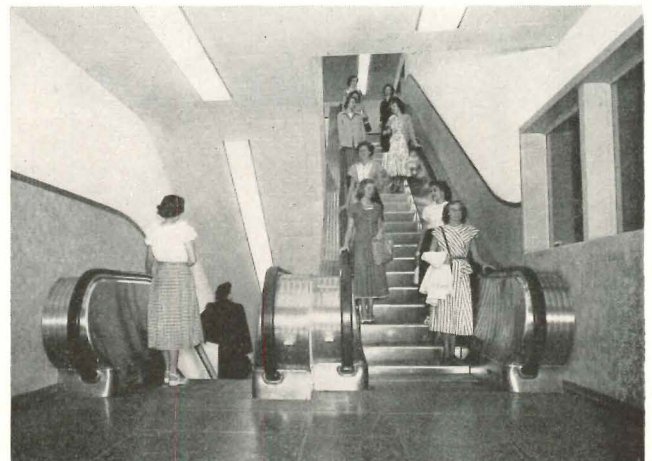
Moving stairways in John Hancock Building run from ground floor to the eighth; elevators serve rest. Cram and Ferguson, Architects
