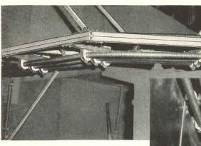
An unusual bracing arrangement utilizes standard Unistrut channel and fittings in attaching the cable-supporting Unistrut framework to wall.
