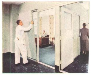
**Maximum mobility** with minimum labor is the result of *I* 30 years experience, all-welded panel prefabrication. WI sections are moved intact, all parts reused.
