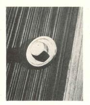
Bolts are retractible so house can be disassembled
