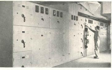
G-E metal-enclosed switchgear handles the incoming 120/208-volt power. The equipment is divided into three sections, two for lighting, one for power. Breakers (cascaded) are of the drawout type for ease of inspection and maintenance.
