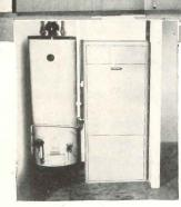
Kew Gardens, Beren, Ohio: One of nearly 100 three bedroom basementless houses designed by Mellenbrook, Foley and Scott and built by Taft and Blockman. The extremely compact Janitrol Winter Air Conditioner uses only a floor space of 22'' x 22'' in the utility room.
