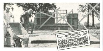
Here's that amazing product that solves one of the biggest troubles with basementless homes . . . cold, clammy floors. Concrete made of Zonolite\* vermiculite aggregate and Portland cement blocks condensation and prevents heat loss.
