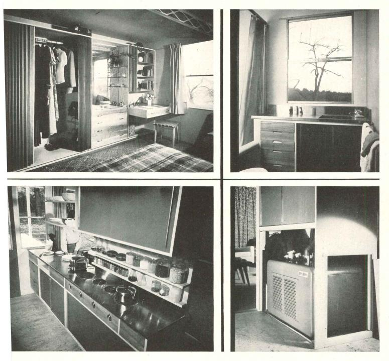
Kitchen, lower left, extremely compact, has recently-developed individual electric cooking units built into stainless steel top, separate oven set at eye level (no stooping), drawer-type refrigerator, wood and tempered hardboard cupboards, total of 103 cu ft of storage. Heater, lower right, is jet-type hot air, oil fired, set in a closet over a utility pit
