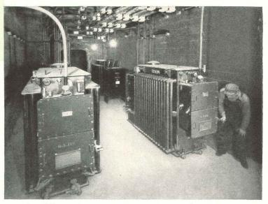
Four G-E network units, rated 500 kva, 12,000-120/208 volts in a Pacific Gas and Electric Company vault serve the building. Macy's 2500-kva load represents one of the largest loads added to PG&E's downtown network in recent years.
