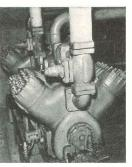
Two Worthington Freon-12 6HF4 Compressors installed in the new annex.
