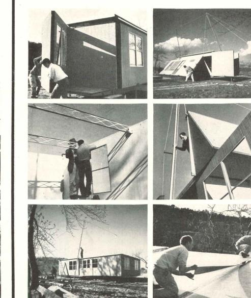
simple boom and one-man winch; center row, placing open-web roof joists and roof panels; bottom row, house nearly erected, roof joints being sealed. Total man hours: for erection, 32; for site preparation, 20
