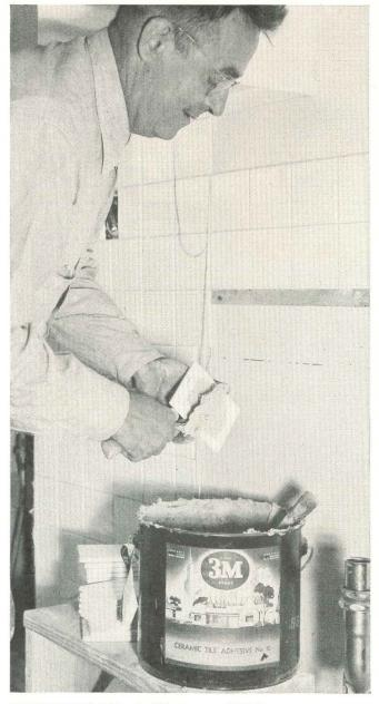
"BUTTERING" TILE at "Hathaway Hills", a quality home project in St. Louis, Mo. Method is recommended when cutting, trimming and fitting is necessary. 3M Ceramic Tile Adhesive can also be used for the faster "floating" method.
