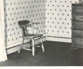
Showing compact installation of Fedders Baseboard Radiation occupying little more space than ordinary wood baseboards.
