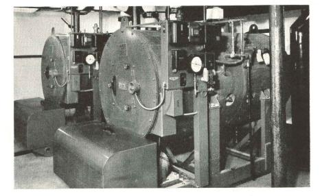
Steam-Pak Generators are built in capacities from 15 H.P. up, for low or high pressure steam or hot water, for light or heavy oil, combination gas and oil or straight gas.
