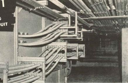
Notice Unistrut's trim steel framework. Note too the Unistrut porcelain and maple clamps that hold the heavy cable and conduit firmly in place.
