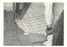
**ECONOMICAL**—Light high-strength — 100,000 psi—steel to take construction abuse. No sag or material waste, concrete placed and finished by common practice on firm stable CORRUFORM.
