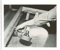
Wiring duct holds fixtures at any point
