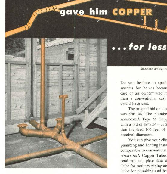
**ANACONDA** Type M Copper Tube and Fittings, in ranchtype residence under construction. Layout for two-bathroom arrangement. Includes 4" soil line; 3" vent stack; waste lines from bath tubs; waste line (riser) for lavatories.
