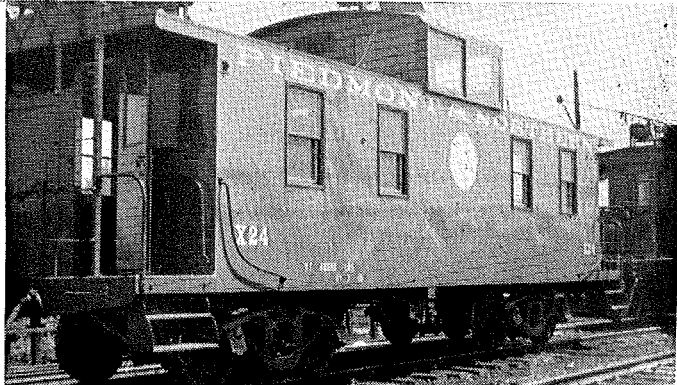
Truscon Double-Hung Steel Windows in Typical Railroad Installation — Piedmont & Northern Railway
