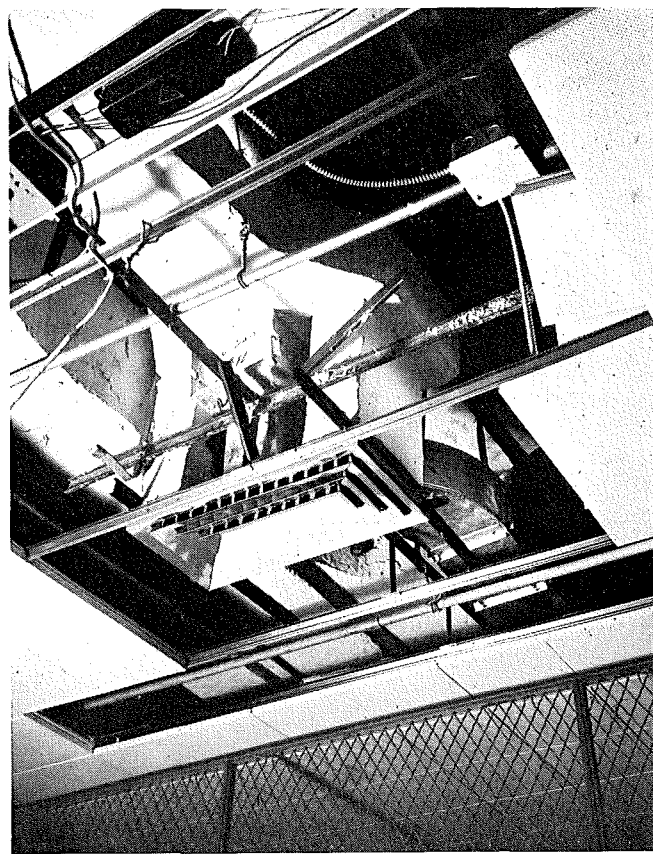
Acoustic ceilings, furred 3 ft., conceal ducts, conduits, etc.
