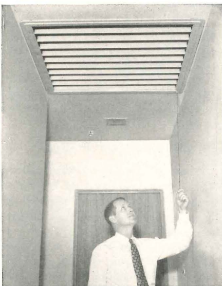
RESULT: cool comfort throughout entire house
