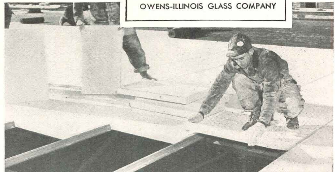
Ease of handling is seen here, as lightweight Kaylo Roof Tile is slipped into place on sub-purlins.
