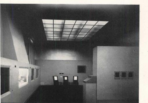
Artificial skylight with light polarizing screen. Note extremely low brightness of ceiling itself relative to that of white paper sheets pinned to backs of chairs
