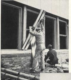
Mullion is screwed to an angle, which is an integral part of the window frame, by stainless steel selftapping screws.
