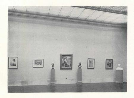
A view of the louvered ceiling in one of the test galleries. This installation gives about three times the light the Museum has at night in other galleries. Color of light is also tested. Upper view shows a test of 6500° K fluorescent lighting on paintings with predominant blues and pastel shades. This lighting is good for them, not so good for reds and greens.
