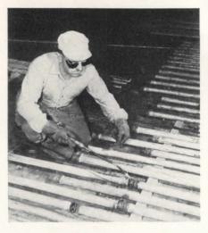
Operator applies silver alloy to braze threadless joint with piping in place
