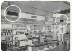
Space is valuable in this modern, compact sandwich shop. Two Janitrol Unit Heaters mounted behind the partition require no floor space.
