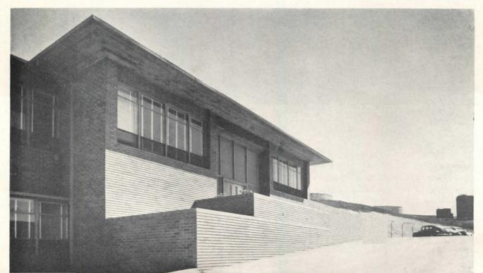
Lobby, recessed of necessity because of the stairs, is opened to daylight with large window panels of corrugated glass
