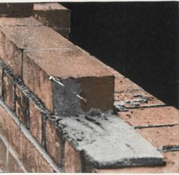
Water entering through the nail holes may travel through connecting voids and find an opening to the inside of the building.
