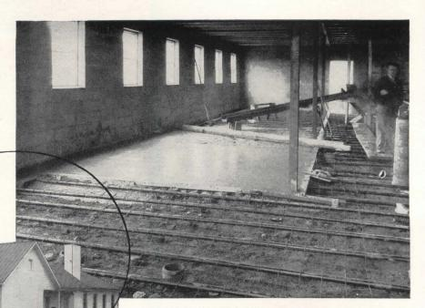
U·S·S NATIONAL STEEL PIPE installed in the floor of a country club locker room to provide radiant heating and eliminate cold floors.
