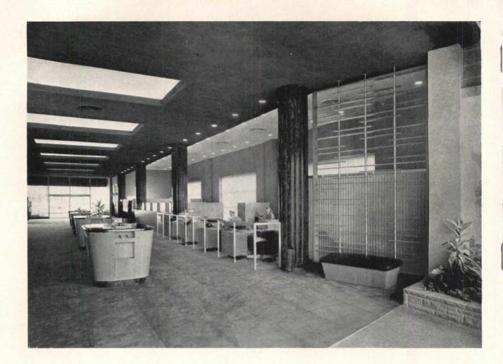
Above: view through the bank from main entrance to parking lot. Columns are green Verde Antique marble. Ceiling is sprayed asbestos to increase acoustical absorption; center portion is 2 ft. lower than side panels, permitting continuous longitudinal fluorescent light troughs. The drop ceiling also has rectangular light troughs, and flush floods are widely used
