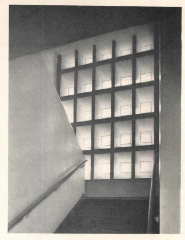
Stair hall windows, a quiet element on the exterior, become a dramatic feature inside, through the simple device of angling the window embrasure to enlarge the opening
