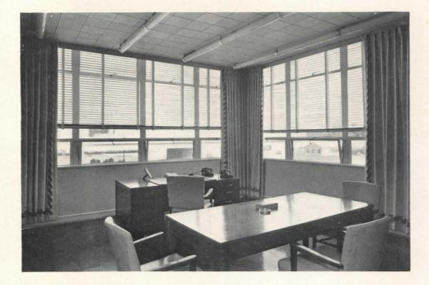
With the exception of the drapes, the manager's office has the typical finish — acoustic tile ceiling, painted plaster walls, asphalt tile flooring, some wood trim in natural finish, and demountable partitions. The structural system is reinforced concrete throughout, with normal column girder and pan floor system, all of which has been reduced to the greatest simplicity to make the building as economical as possible
