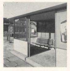
This small island building—also prefabricated of enameled iron panels serves as a sheltered waiting room, with neatly designed wood-slat benches inside
