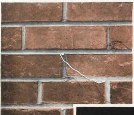
Nail holes are a frequent cause of leaks in masonry walls. If these holes happen to connect with voids in the head joints, water may enter, and then travel through connecting voids in the bed joint until it finds an outlet on the inside of the wall. When a nail or line pin is used, the hole should be plugged with mortar immediately after the nail is removed.
