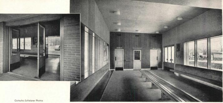
Although the south-bound platform building represents an alteration rather than a new design, its entire character has been completely "revamped." All interior details, such as wall-paneling, cantilevered seats, terrazzo floors, and wide glass areas are impressive for their simplicity and ease of maintenance. The lettering within the station—an important point in railroad design—is distinguished for its clarity
