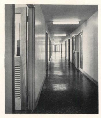
Manager's office, right, shows standard office interior — acoustic tile ceiling, asphalt tile floor, painted plaster walls This corridor photograph could have been taken in either of the two office buildings, as both interiors are identical. Ceilings are furred down for air conditioning ducts; floors, asphalt tile
