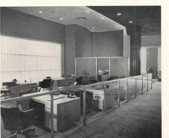
The officers' section (left) is separated from the public area by a plate glass railing. Corrugated glass screens the conference room Lighting has been carefully worked out to maintain approximately 35 footcandles at counter height for the critical areas such as desks, counters and tellers' cages. Detail of light cove at right
