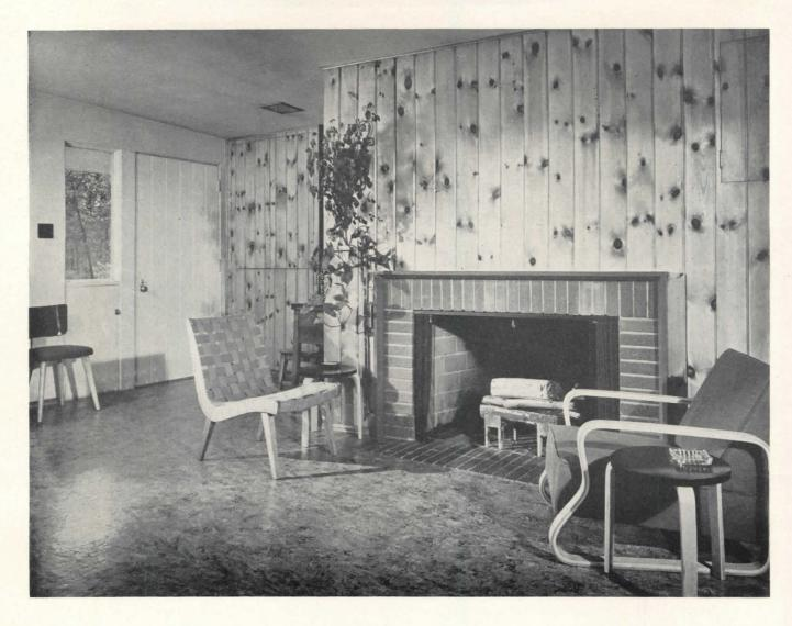
Above: the fireplace wall in the living room is of knotty pine, contains unusual storage facilities; main entrance is at left. All windows are fixed sash except for kitchen casements, and ventilation is controlled by louvers beneath the windows and a fan and duct system. Floors are linoleum covered, lighting is fluorescent
