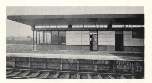
The prefabricated Marsh Lane Station again utilizes the raised cantilever canopy, which admits clerestory lighting to the platform. The lettering seems far too small for practical legibility—a common fault of British stations. Plans below show the flexibility of this prefabrication system
