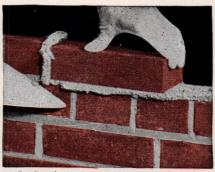
So that the mortar cozes out at the top of the head joint.
