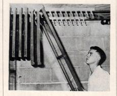
Brackets fastened to overhead joists store up to 21 storm window and screen sashes, protecting them from damp floors
