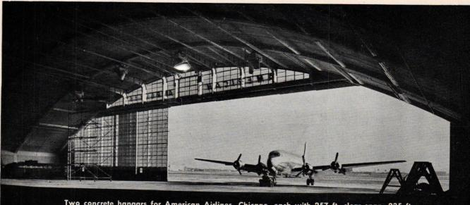
Two concrete hangars for American Airlines, Chicago, each with 257 ft. clear span, 235 ft. door opening, and an acre of unobstructed floor space, provide elbow room for largest planes.
