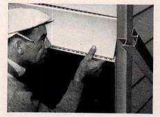
HERE IS THE ONLY metal siding with a preformed curved surface. The plain upper edge of each piece slips into the slotted lower edge of the piece above. Nailing down the lower edge produces a strong tension. Result: A rigid, weatherproof joint. Work is speeded by pre-punched holes. Money is saved because only half the usual number of nails are needed and no wood sheathing is required!
