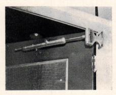
Door closer uses brake lining principle
