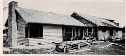
**KAISER ALUMINUM** clapboard Siding can't be weakened or disfigured by knots, splits or sawing scars. It can't rot, warp, rust or crack. And a zinc chromate prime coat applied at the mill readies it for
