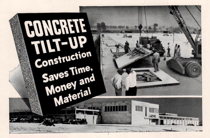
**TILT-UP,** the fast, modern and economical method of concrete construction was used in building the Luthe Hardware Company warehouse in Des Moines, Iowa—a structure with more than two acres of floor space.
