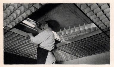
Easy-to-install Alumigrid units are 4-foot square and weigh only 10 pounds. Supported by a framework of aluminum rails, these units are easily lifted aside for re-lamping or maintenance work on ceiling elements above.
