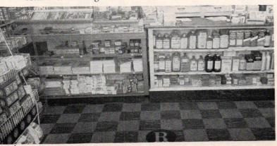
This Glendale, California Rexall outlet (below left) acquired the "new look" with a new, marbleized asphalt tile floor in a smart, gray-green checkerboard pattern. To direct store traffic to the prescription department, an inexpensive asphalt tile insert was used.
