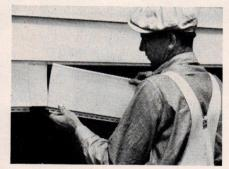
**TIGHT, CLEAN-CUT** butt-joints are easily made with back-up plates available with the new siding. Paint finishes completely conceal the joints. Notice, too, that all nails are hidden. The concave surface makes beautiful, 3/4" deep shadow lines and eliminates oil can sheen, waves and buckles. The new material can't be damaged by rats or insects either, and never needs the usual kind of maintenance.
