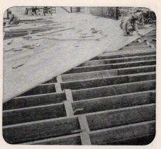
3. Wood used in or near the ground open to attack by termites.
