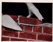
So there will be more than enough mortar to fill the joint completely when the next brick is pushed into place.
