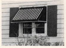
Awning louvers, adjusted by a control arm, permit any degree of light and ventilation
