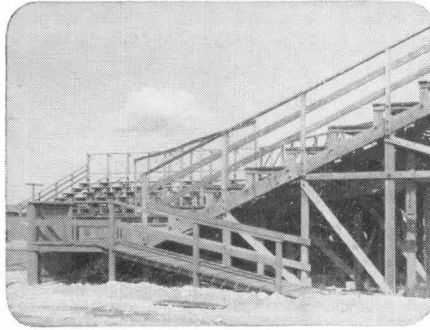
1. Ground moisture and rain held in joints etc., of outdoor structures.
