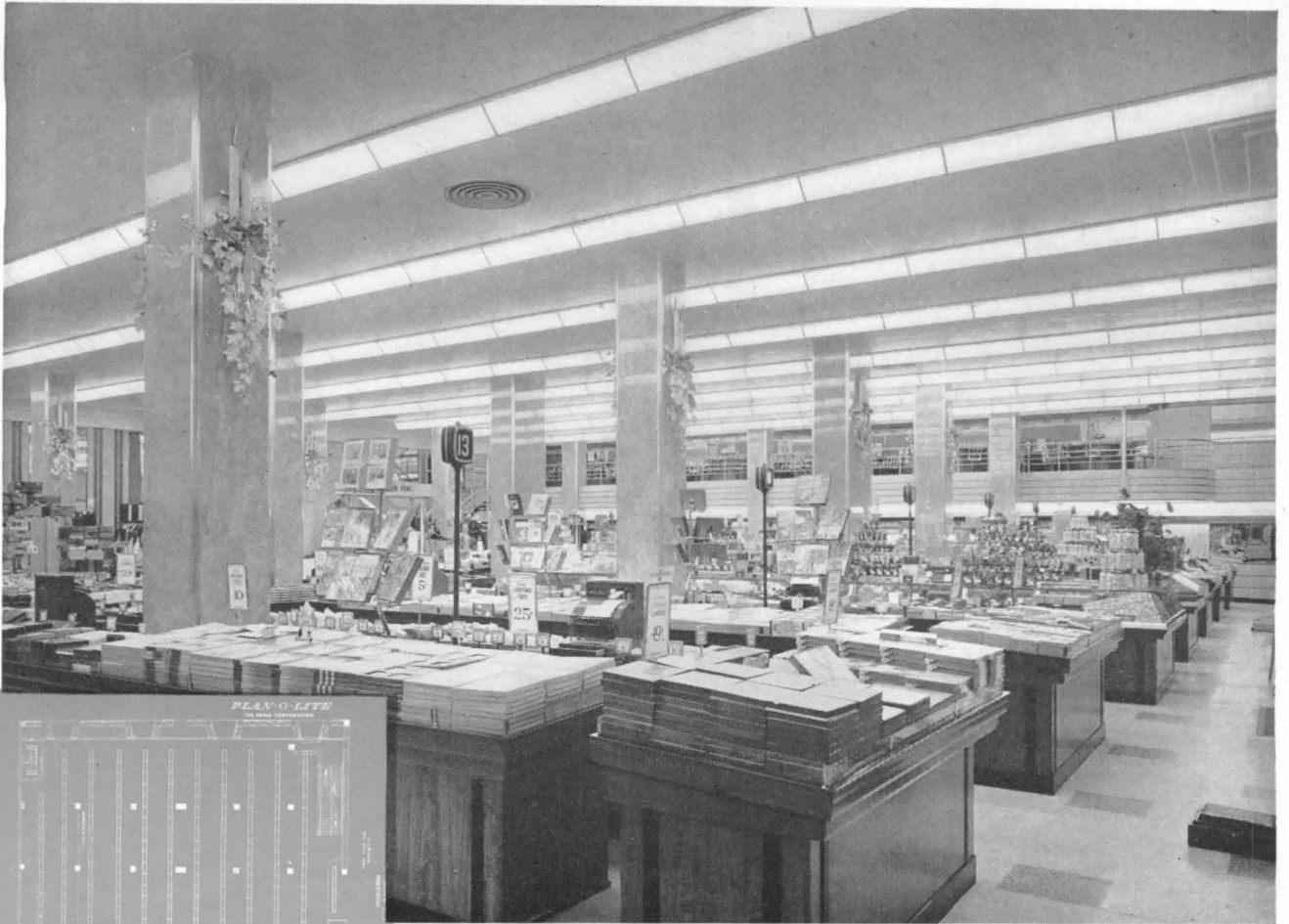
Main Selling Area, F. W. Woolworth Co., Detroit, Mich. This entire store is illuminated with over 3000 feet of L-I-N-O-L-I-T-E No. 7348, ceiling mounted in continuous rows. Similarity of the entire system tends to integrate all floors into one large selling area. Approximately 45 foot candles average maintained.
