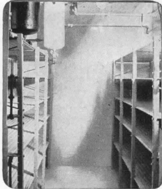
Quick-freezer Has Shelf Plates Held at -15° to -20° F.
