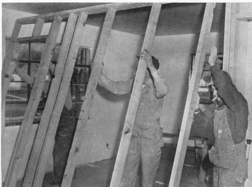
Above and below: in various tests partitions were tipped up before gypsum board was applied, and with gypsum board on one side only; the 4 by 12 size saved on taped joints
