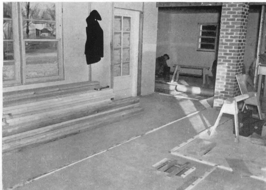
Above and below: finished flooring is laid before partitions are erected, and protected with one layer of wrapping paper and one of sisalkraft, held down by batten strips
