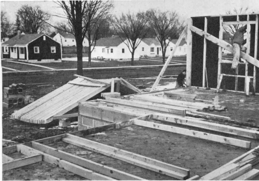
Above: walls being assembled on subfloor, one wall in place, roof trusses in background
