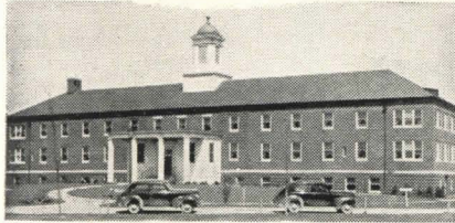
CENTRAL MICHIGAN COMMUNITY HOSPITAL Mt. Pleasant, Michigan. J. Walter Leonard, Chairman, Hospital Board. Built 1942. Architect: James Gamble Rogers, Inc., New York. Consulting Engineer: Jaros, Baum & Bolles, New York. Heating Contractor: A. W. Eurich, Bay City, Michigan.
