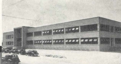
Truscon Intermediate Projected Windows installed in the Eight-by-Six-Foot Supersonic Tunnel office building at the Flight Propulsion Research Laboratory of the National Advisory Committee for Aeronautics, Cleveland, O.
