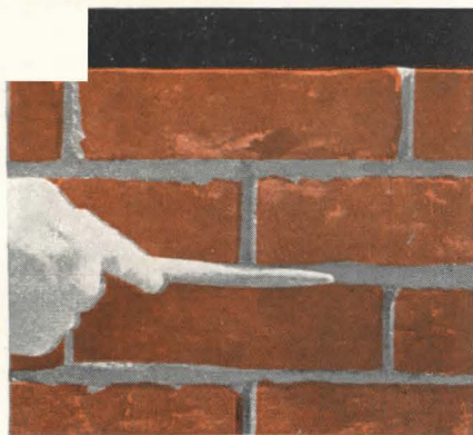
As an alternate for backplastering, the joints on the back of the face brick may be tooled to give a concave finish.
