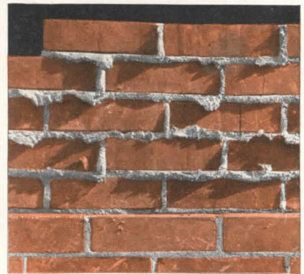
Before backplastering, however, all mortar joints should be cut flush. Parging should not be attempted over protruding mortar joints.
