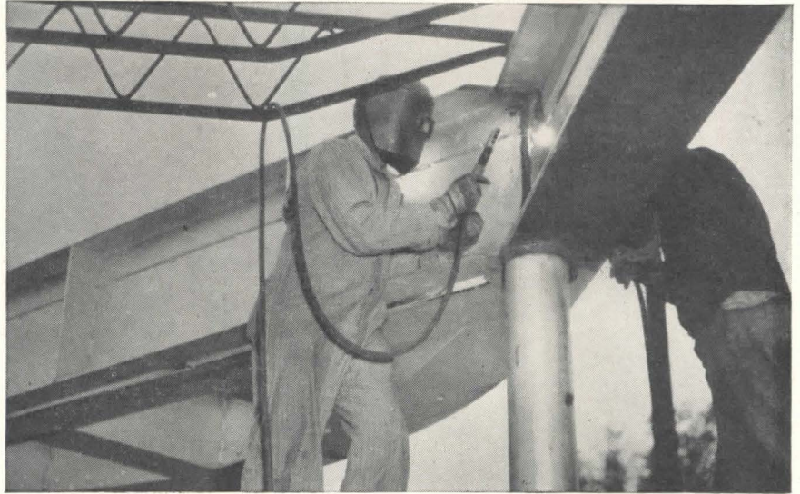
Fig. 2. Two welders weld heavy beams simultaneously to avoid distortion.
