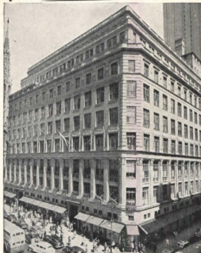
SAKS & COMPANY, Fifth Avenue, New York, N.Y. Built 1924. Architect: Starrett and Van Vleck. Heating Contractor for original installation: Gillis and Geoghegan. Heating Modernization 1944 by Contractor Thomas J. Dorsey, Inc.
