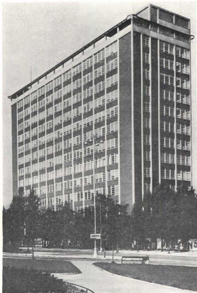
Above, dormitories for student workers range in tiers up the hillside fairly close to the central plaza (shown in the center above). Below, the Administration Building, 1938, noteworthy for its straight-forward expression of the standardized construction used for all major buildings, as described in text
