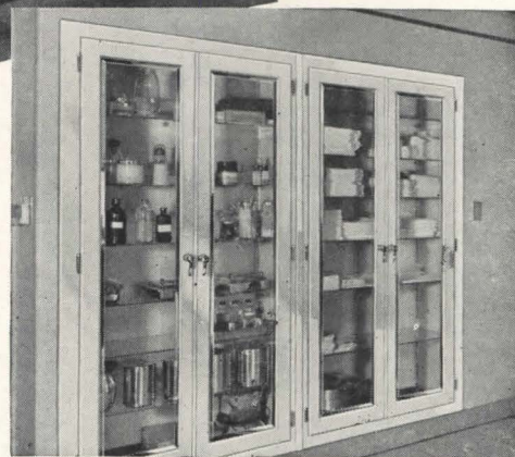
Recessed supply cabinet in septic operating room
