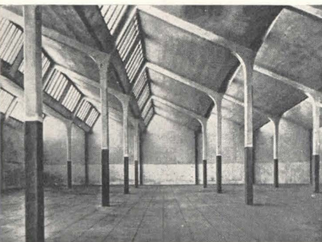
Benet factory Barcelona, Spain Robert Maillart engineer (1924)
