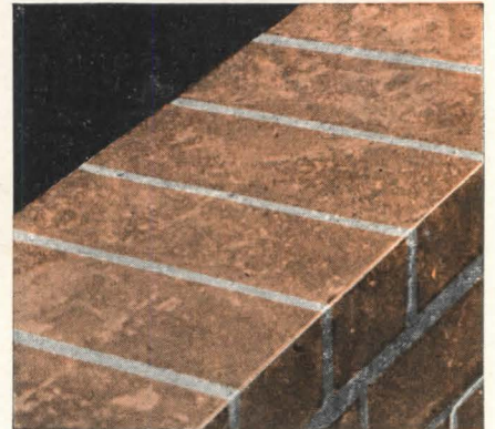
This completely fills the joint.
