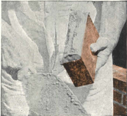
Mortar should be spread over the entire side of the header brick before it is placed on the wall.
