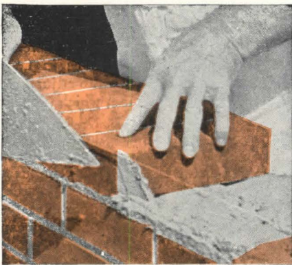
When a dab of mortar is spotted on one corner of the brick,
