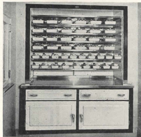
Recessed cabinet in maternity department. Upper section open and fitted with adjustable stainless steel shelves for holding mothers' treatment trays.
