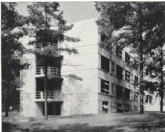
Piedmont Sanatorium, Burkeville, Va., is one of several concrete hospitals designed by Williams, Coile and Pipino, Newport News, Va., John T. Wilson Co., Richmond, Contractor.
