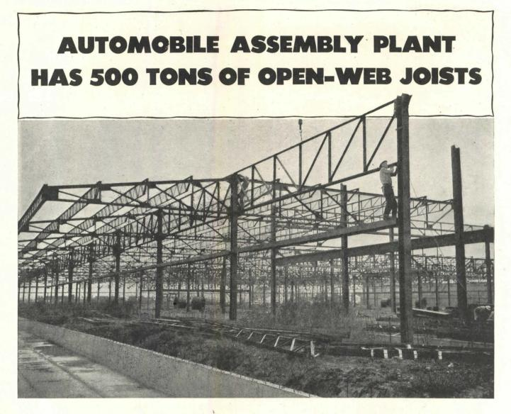
Shown under construction at Los Angeles, California, is the huge Lincoln-Mercury assembly plant of the Ford Motor Co. Designed by Harry R. Miller, and erected by William P. Neil Company, both of Los Angeles, the L-shaped one- and two-story structure is about 840 ft in length, and 600 ft wide. To permit large expanses of clear floor space with a minimum of columns and thus facilitate manufacturing and assembly operations, 500 tons of Bethlehem Longspan Joists were used.
