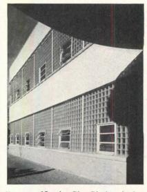
Harmony of Insulux Glass Block and other building materials is readily seen here. Small clear windows, set in the panels with standard frames, provide vision out and ventilation.
