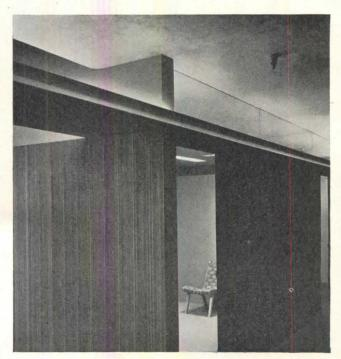
To allay possible claustrophobiac sensations in the minimal office spaces, partitions are topped with glass transoms to give ceiling spread. In photo above, striated plywood panel flanks corridor leading to main sales area. Lighting along top of front partition is by means of three continuous fluorescent lines, with reflector; there are four lines over entrance to the corridor
