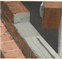
Then the excess mortar will fill the furrow and insure full bed joints.
