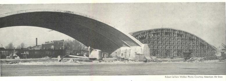
Concrete hangars seen above are in Chicago for American Air Lines, by Whitney and Ammann, engineers. Slab is on the neutral axis of the ribs, creating an economical, more flexible structure. Buttress area provides shop space. (Span, 257 ft.) Cantilever trusses seen at right (**E**, steel, **F**, concrete) are short in hemselves but allow endless lateral spans
