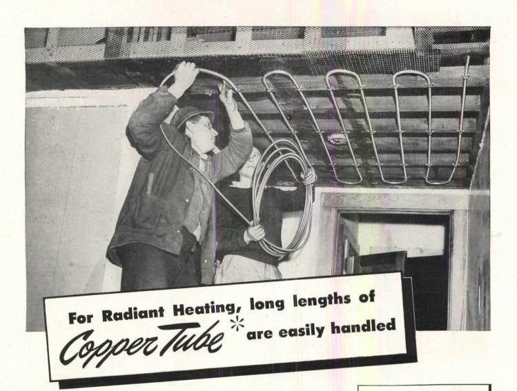
In radiant heating, the light weight of Chase Copper Tube is an outstanding installation advantage—particularly for ceiling mounting.
