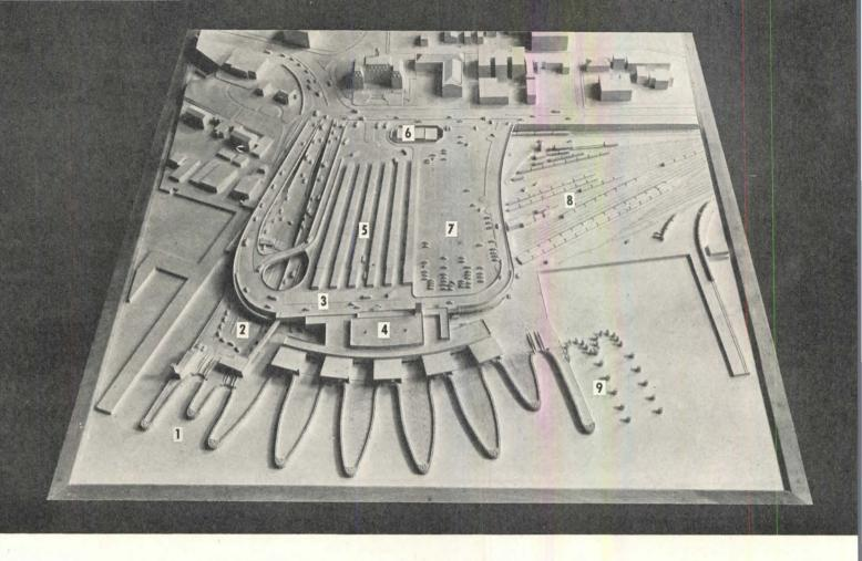
Key to photos of model, above and opposite page: (1) slips and (2) vehicle lanes for Brooklyn ferries; (3) taxi, private car and bus viaduct; (4) roof of terminal; (5) bus loading and unloading platforms; (6) transformer station; (7) parking space for 500–600 cars; (8) railroad yards; (9) lay-up and repair slips; (10) vehicle lanes for Manhattanbound ferries; (11) railroad terminal
