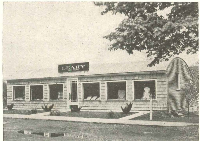
(Above) Left: Auditorium of small movie theater at Aurora, Colo., is a 40-ft. wide Quonset. Right: Cut-away front and wood shingles disguise the Quonset origin of this store building at Sayre, Pa. (Below) Left: 20-ft. Quonset can be converted into a cattle barn. Center: Multi-arch construction provides roomy industrial shop. Right: Supermarket in Greenville, Mich., is adapted from a Quonset "40"
