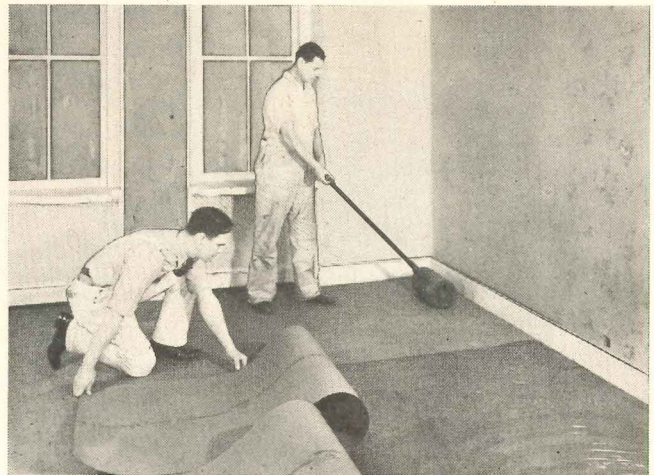
Lining felt should be installed with the strips placed at right angles to the floor boards. It should be cut to fit accurately with a minimum of seams. The felt should be firmly bonded to the adhesive-covered subfloor by rolling out from the center in all directions.
