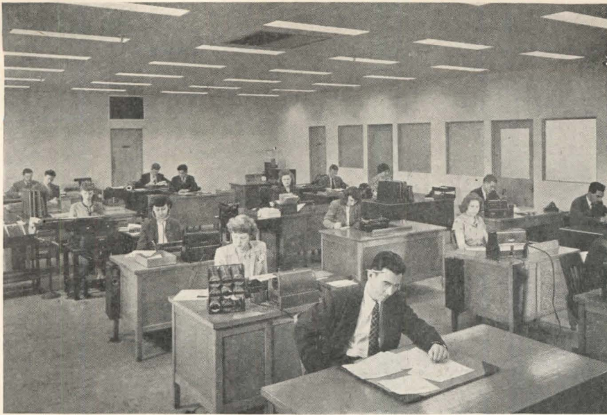
Sound-treated ceiling and recessed fluorescent lighting of 35 footcandles, plus air conditioning, make for comfortable working conditions in the office portion. Sprinkler pipes are concealed in ceiling
