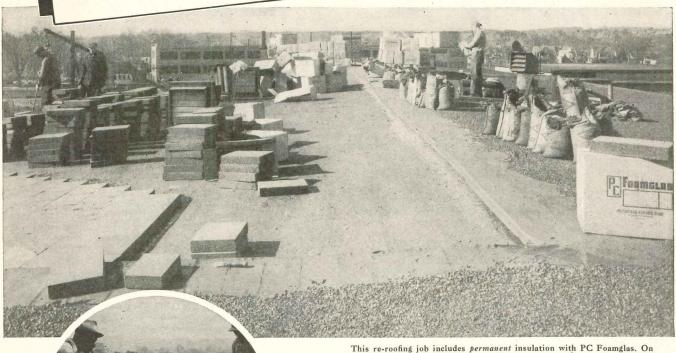
This re-roofing job includes permanent insulation with PC Foamglas. On new construction and on modernization projects on all sorts of plants, PC Foamglas Insulation has licked the toughest jobs. An impervious, inorganic, cellular material, PC Foamglas, retains its insulating value—indefinitely.
