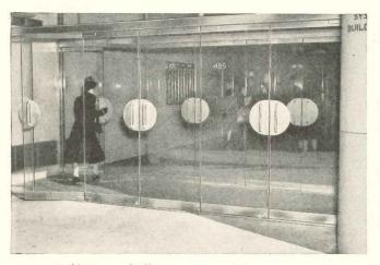
Architects are finding many new design possibilities for entrances since the development of Herculite Tempered Plate Glass. Sturdy, handsome doors of crystal-clear Herculite help to create entrances that are distinctive and impressive. In the application shown, inner and outer doors are of Herculite, with an over-door panel of lustrous Polished Plate Glass.
