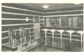
Sanitation in public building washrooms is often determined by the material used for walls and partitions. Carrara Structural Glass is a modern material that permanently retains its polished beauty and excellent sanitary properties. It is easy to keep clean. It will not check, craze, stain, nor fade. It is impervious to water and pencil marks. Ten colors of Carrara are available to help the architect achieve attractive washroom designs. Architects: Marr & Holman.
