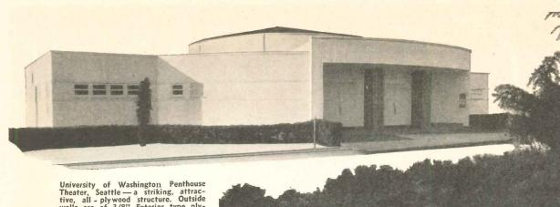
University of Washington Penthouse Theater, Seattle—a striking, attrac-tive, all - plywood structure. Outside walls are of 3/8" Exterior type ply-wood over 3/8" plywood sheathing.
