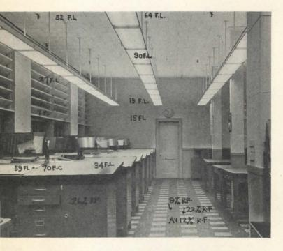
Below, same room by day. Brightest area, the window louvers, is held down close to ratio of 3 with work. Inner wall is in need of supplementary artificial lighting to keep brightness even
