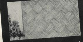
This design illustrates one use of Weldtex, the popular striated Weldwood paneling. The striations lend an attractive third-dimensional effect to the panel, and likewise conceal joints and nail holes.
