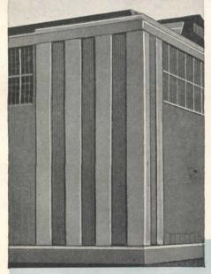
Typical Exterior, Mahon Steel Deck Sidewall Construction. Pilaster effect is obtained by reversing Deck Plates so that ribs face in, as opposed to remainder of wall where ribs face out.
