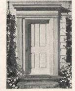
Curtis Entrance C-1730 recalls many fine doorways found in Connecticut and Massachu-setts. Note the entablature with its bowed face, dentil course and pilaster beading. H. Roy Kelley, Architect.
