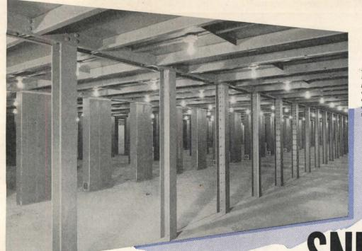
Showing the essential construction stripped of stacks and partitions. Steel plate floor and structural stack columns are designed, fabricated, and spaced accurately to bookstack tolerances to accommodate the equipment shown in the floor plan.
