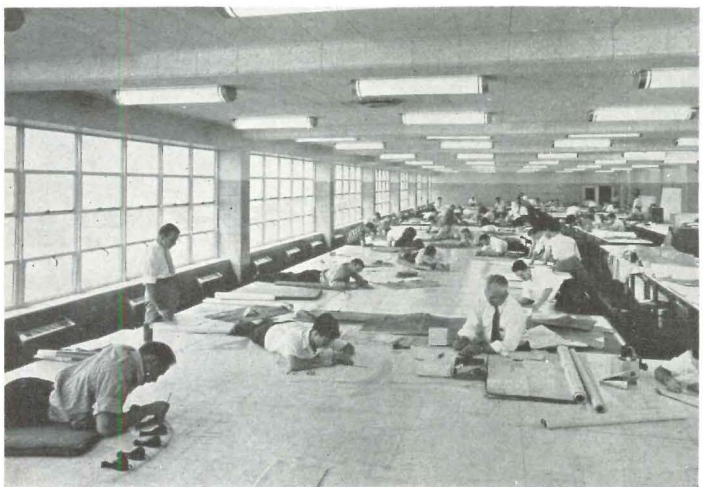
The new light sources, with lower brightness contrast, are rapidly making possible the high-level even kind of illumination formerly dependent on daylight. Both solutions above are clean. White paper is a splendid diffuser of light
