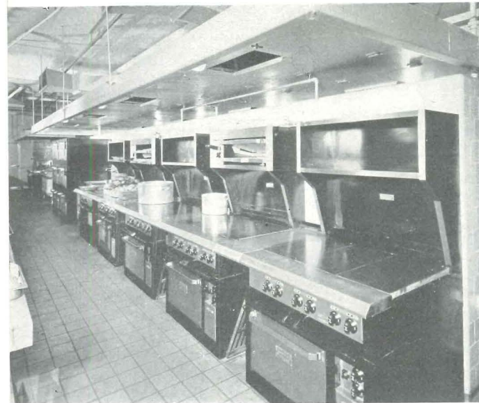
Carefully vented battery of ranges in the view below is to be seen again in the background of the view above. The size of the plant kitchen depends on the size of the total work force and not, like the dining rooms, on the largest shift
