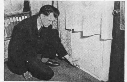
Hollow cast iron "radiant baseboard"
