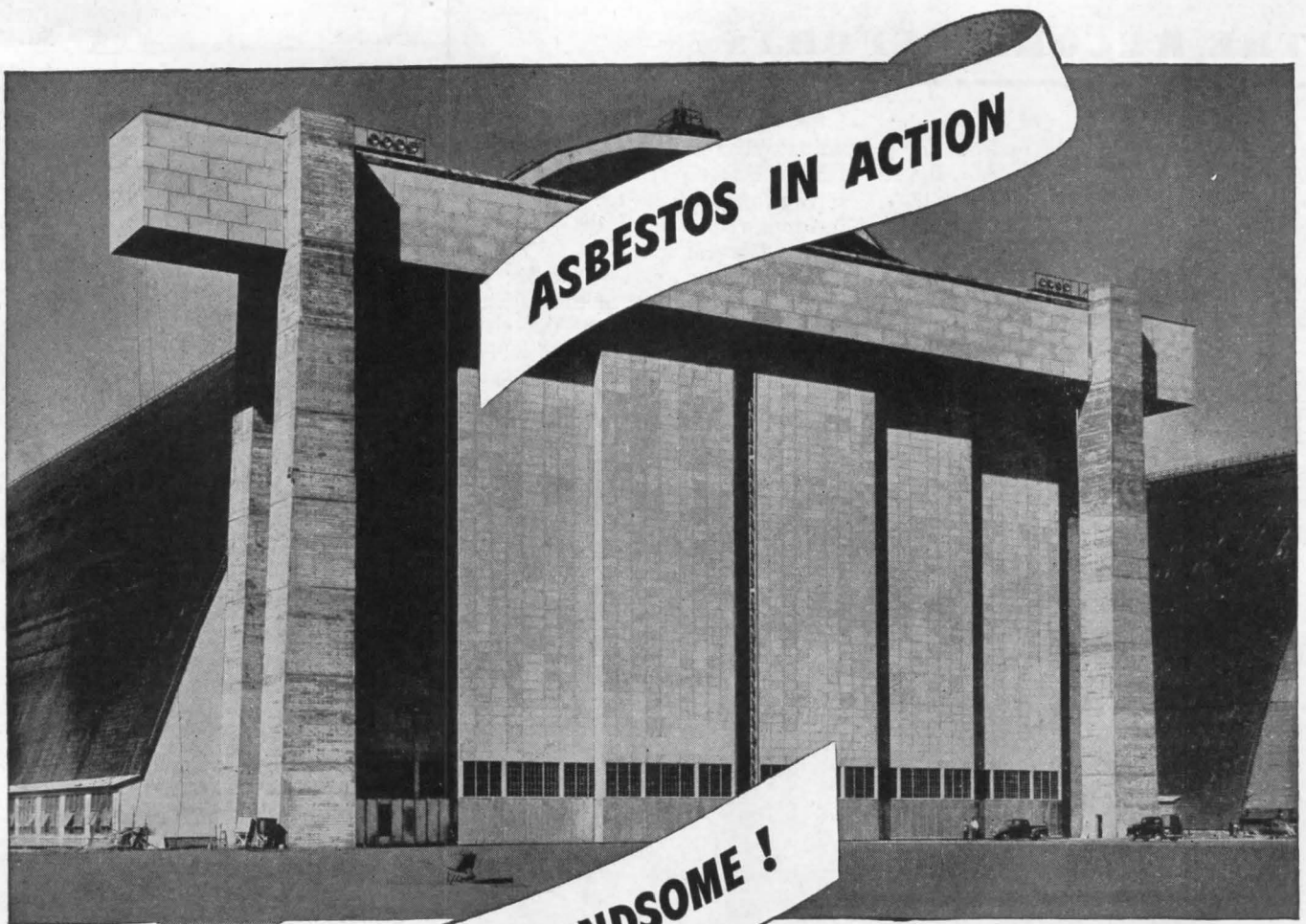
Designed, built and erected by Byrne Doors, Inc., Detroit. Apac Sheathing installed by the Faulkner Construction Company. (Official U. S. Navy photograph.)
