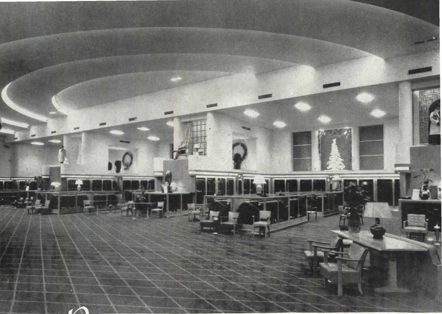
INTERIOR OF THE BOND STORE, 45TH ST. & BROADWAY, N.Y.
