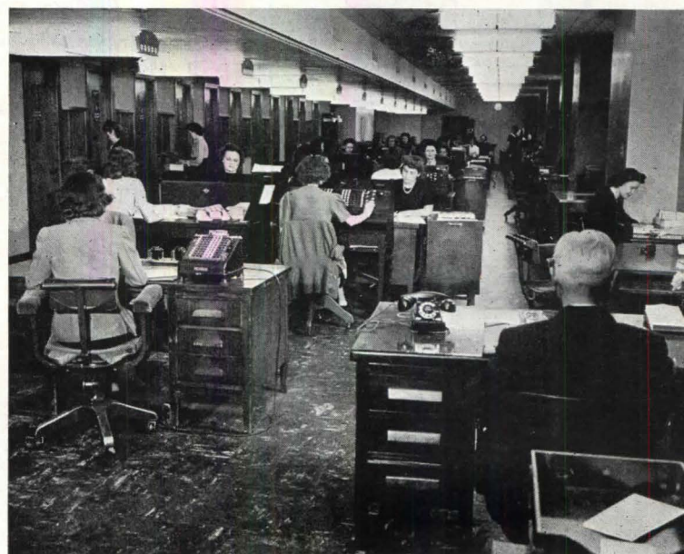
Bank offices on the third floor, like the rest of the building, are completely air conditioned. Ceilings are of acoustic tile, lighting fluorescent. All flooring is asphalt tile
