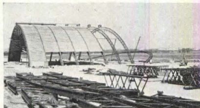
ARMCO hangar being built at Washington National Airport as ATC headquarters
