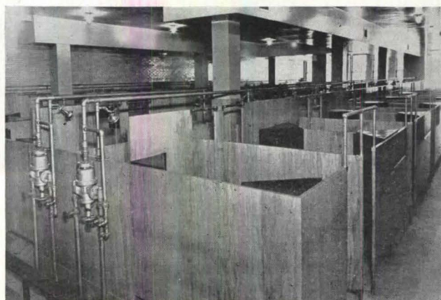
Girls' gym lockers fitted into individual dressing rooms
