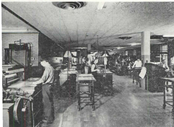
The composing room, wood floors acoustic ceiling
