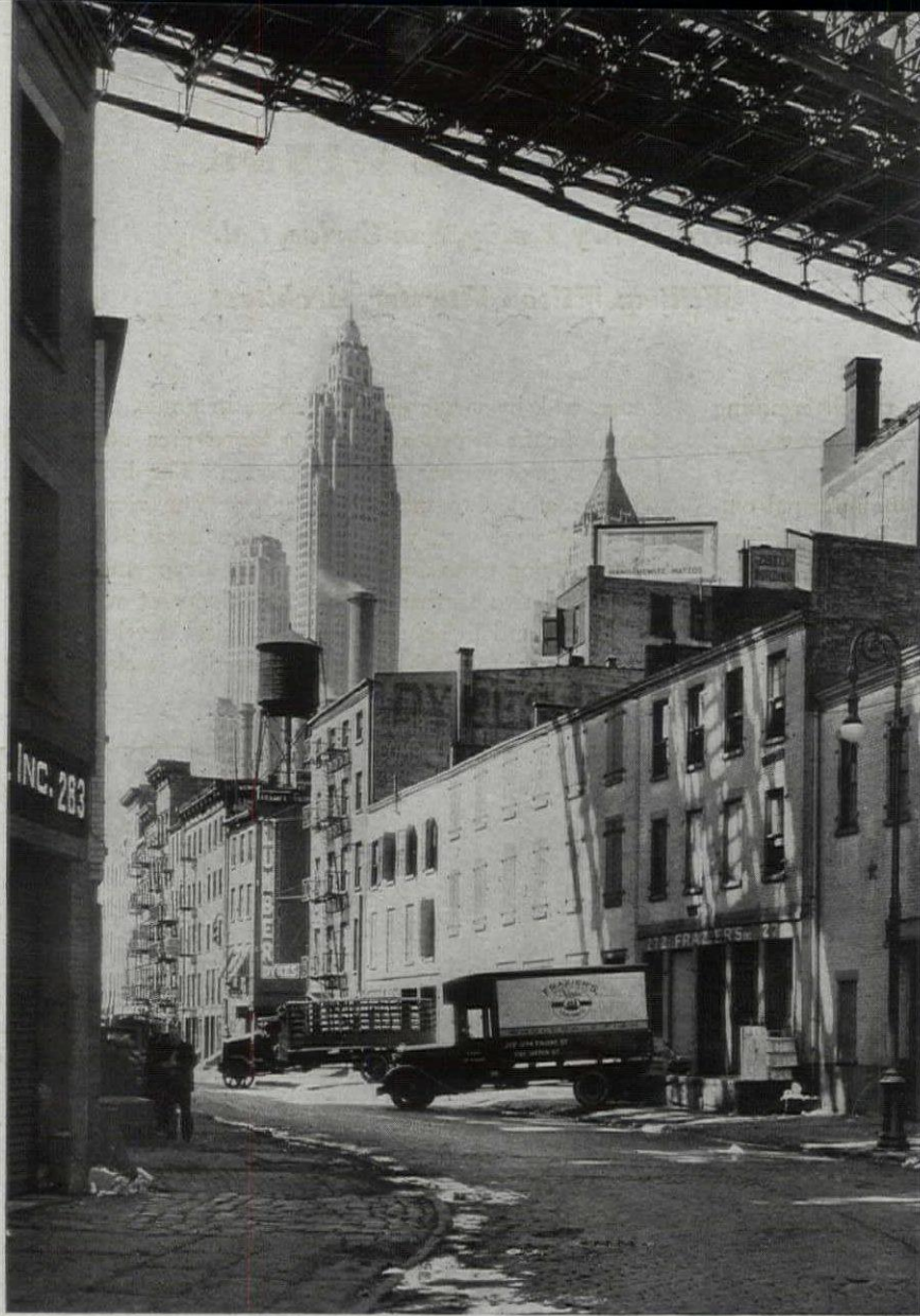
Beneath the Elevated on New York's Pearl Street. Here are seen obsolete buildings on the original small plots of land. These are used largely for warehousing, despite inefficient and wasteful operating costs. Even though the location is close to the water front, rents are low because of depreciation of properties. The most economical solution, says the author, would be a voluntary agreement of owners to pool interests for replanning and rebuilding on a scale suitable for modern uses. The New York Urban Redevelopment Law of 1941 was designed to make such a project possible.
