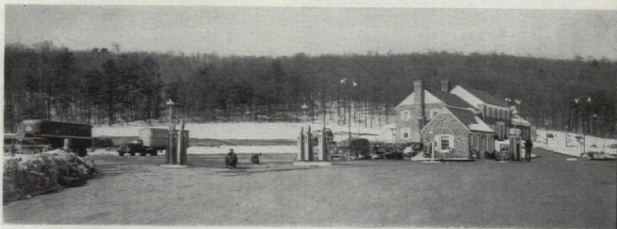
Midway includes Howard Johnson restaurant, also truckers' lunch and dormitories. Trucks enter at right, swing far to rear, emerge at same service station as passenger cars
