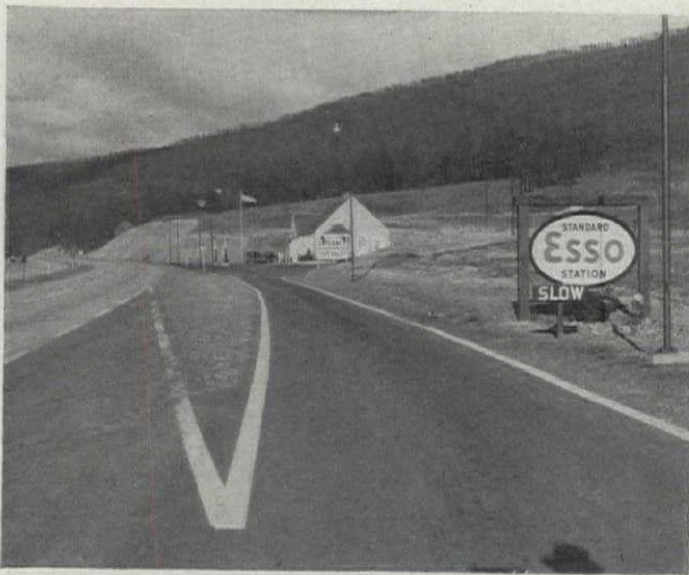
The V of a 1,200-ft. approach lane of a high-speed highway station (Penn Turnpike). See text, under "Approaches"
