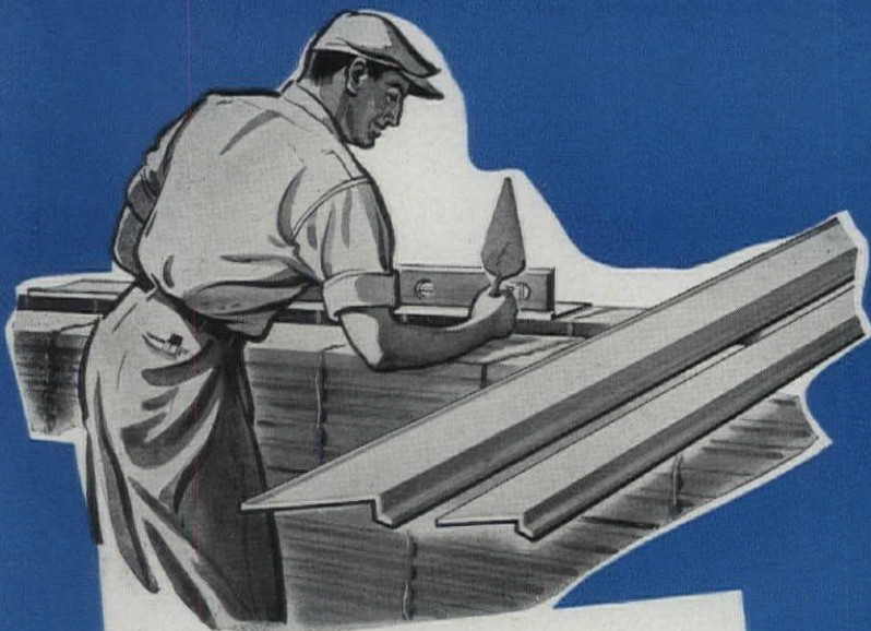
Aluminum sill used with double-hung aluminum window; equally adaptable to a wood window.
