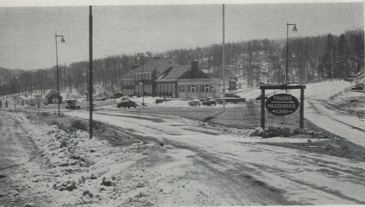
At the Midway Station, truck and passenger-car approaches are separated. At left, station plan (a smaller parking area is across the turnpike); across-page, main building plans
