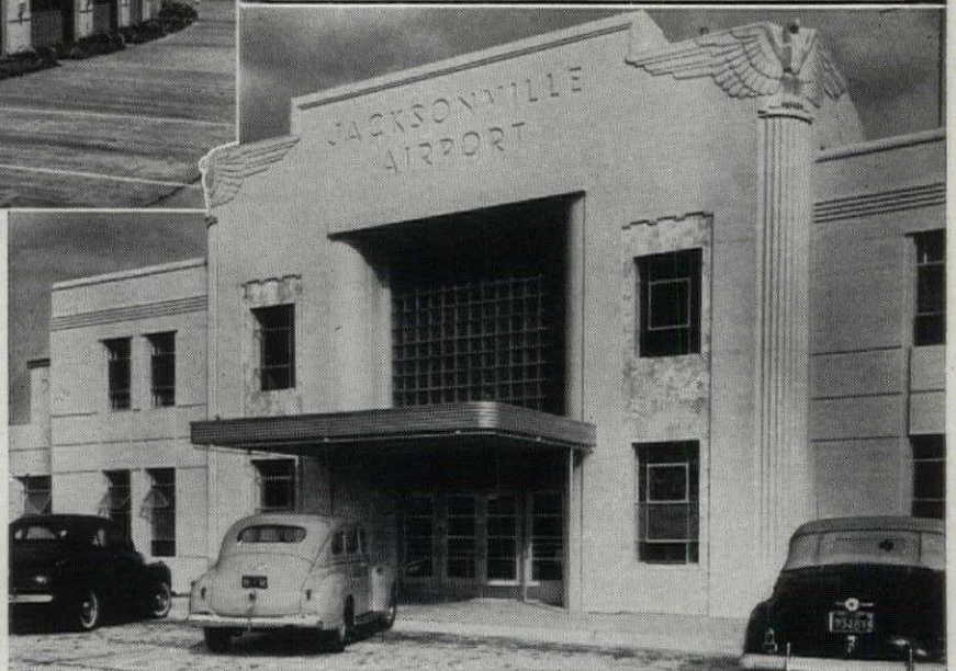
Below—Decorative details on administration building at Jacksonville, Fla., Municipal Airport are an integral part of the architectural concrete structure designed by Jefferson D. Powell, Jacksonville architect.
