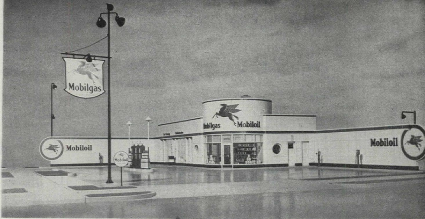
Advanced station model in current use; Frederick Frost, architect. The "drum" shape is a trademark. Porcelain enamel finish, standardized elements, efficient arrangement, good screening
