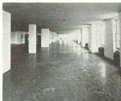
Asphalt tile flooring was laid solid from wall to wall in Mercantile Bank Building, Dallas, before partitions were installed
