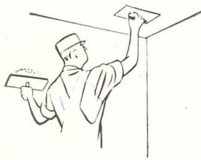
ACOUSTICAL PLASTER FINISH
