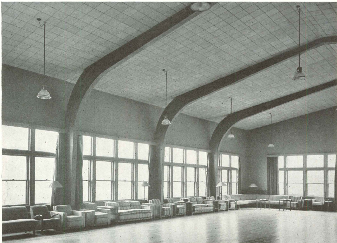
Graceful laminated arches give character to the large hall
