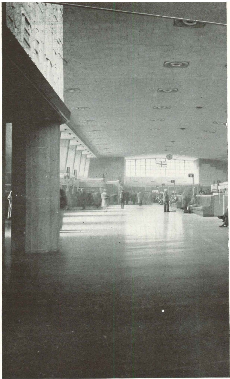
The large view above, and small views across the bottom of both pages, show waiting-room facilities. Above, the unobstructed view across concourse from the waiting room end
