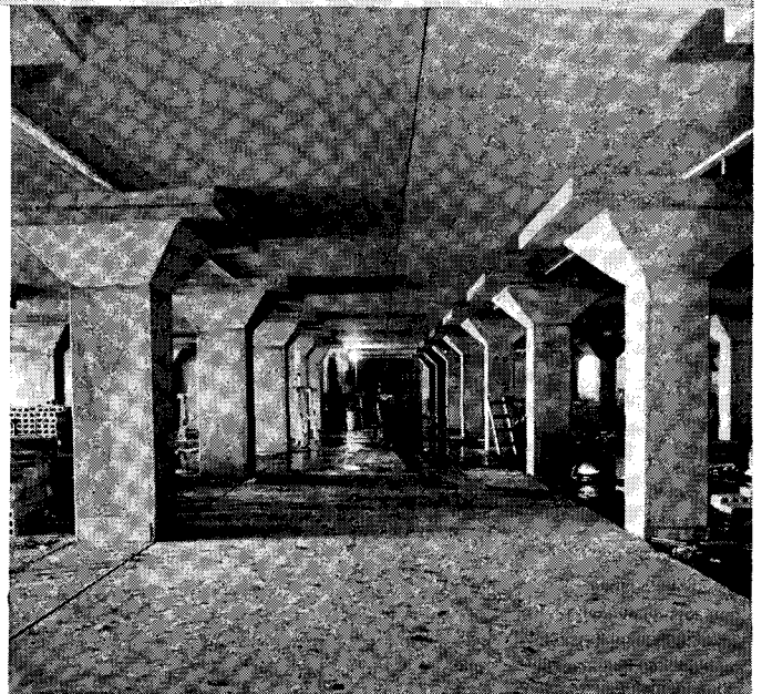
All-concrete Administration Building of arsenal in middle west. Designed by U. S. Engineer Office. Priester Const. Co., Davenport, Iowa, contractor.
