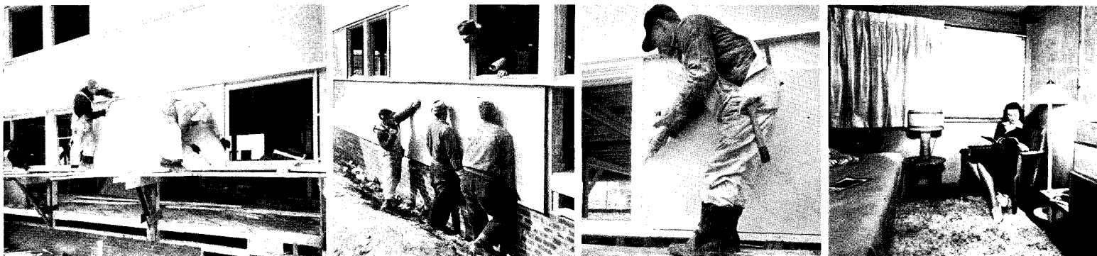
7,000 girls. Outer walls and partitions are inch-and-a-half Cemestoboard (Celotex) nailed to a structural frame of precut members
