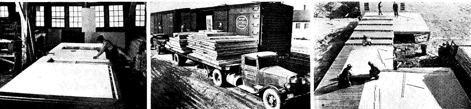
Sheets large enough for an entire wall provide unbroken surfaces in the system of The Upson Company. These pictures show the whole-wall
