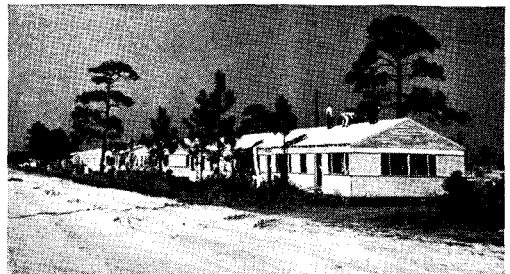
Here is one section of Cemesto housing units which comprise one Florida development.
