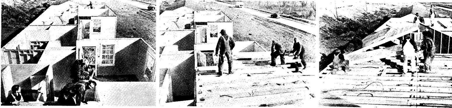
panels being built in a plant at North Tonawanda, N. Y., trucked to box cars, and being assembled in Dayton, Ohio, in a war housing project
