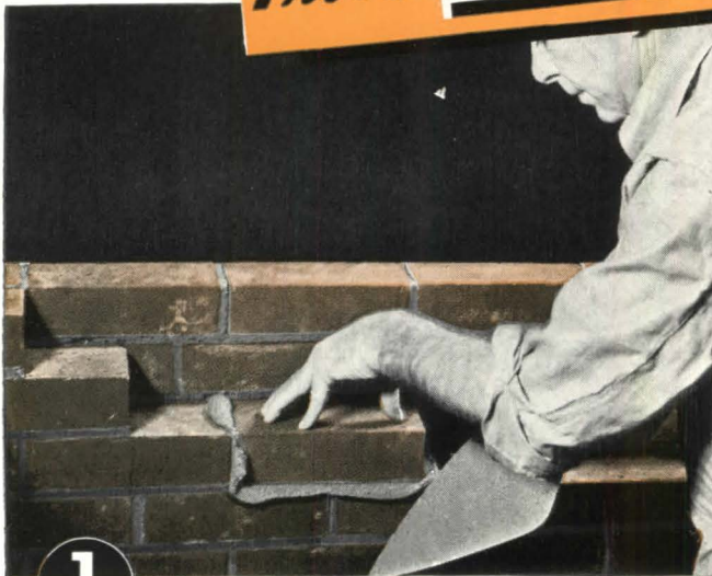
1 Take some Brixment mortar and some 50-50 lime and cement mortar. Try shoving a full head-joint with each mortar. You'll find that with the Brixment mortar
