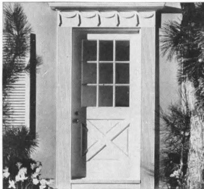
Entrance C-1765, Cameron Clark, Architect. Design of famous architects—plus Curtis production—makes such entrances available.
