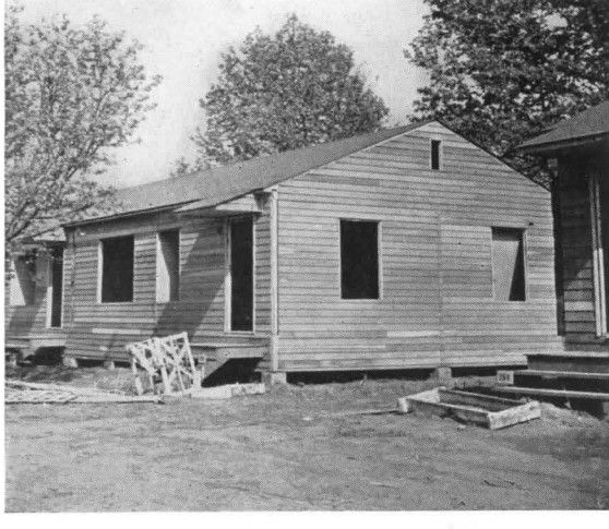
F 1. A row of houses, nearing completion; the siding is redwood. 2. A creosote mixture is sprayed on exterior walls with a spray gun and com-
