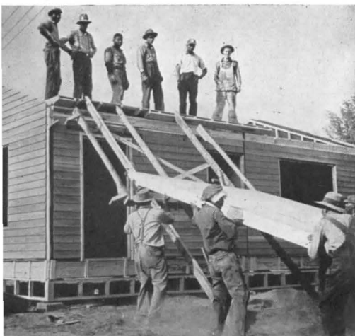
1. Ceiling panels and roof sections are raised by means of a greased skid. 2. Roof pitch is achieved without trusses by propping two sections against
