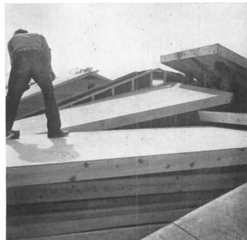
1. Ceiling panels and roof sections are raised by means of a greased skid. 2. Roof pitch is achieved without trusses by propping two sections against
