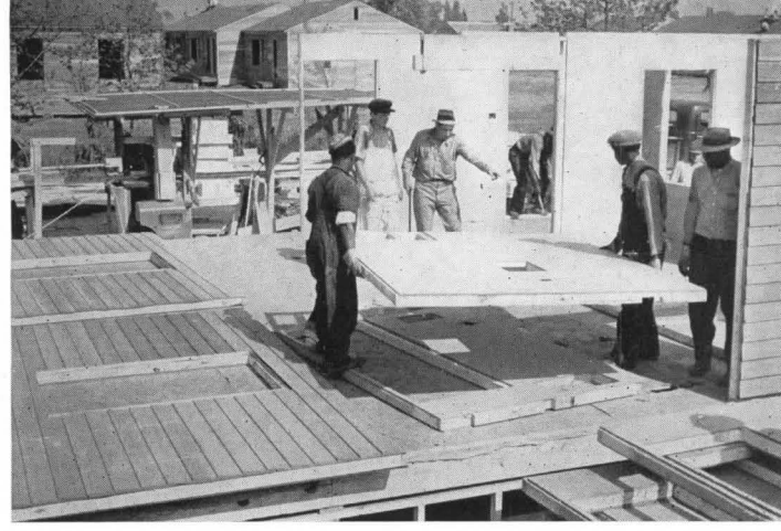
D 1. Floor panels are raised on the underpinning. As soon as floors are laid, heavy building paper is laid over them to protect them during re-
