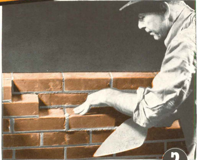
(1), it is much easier to shove the brick accurately into place, with a full head-joint, than it is to do the same thing with the other mortar (2).
