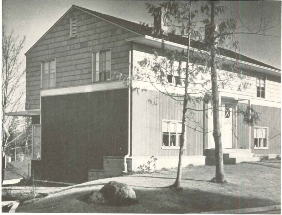
Two-story hillside unit, with entrance between floors
