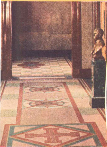
terrazzo floor, made with Atlas White cement, in City Hall and Auditorium, Montgomery, Alabama. Architect, Frank W. Lockwood; General Contractor, Algernon Blair, both of Montgomery. Sub-contractor, Fornara Tile & Terrazzo Company, Atlanta.
