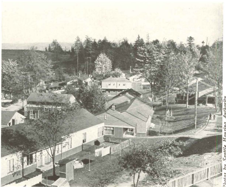
Photos by Seattle Housing Authority
