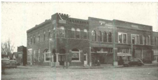
Starting in the building at the right, fire gutted the next two structures (see photo below), but a J-M Asbestos Roof saved the bank on the corner.
