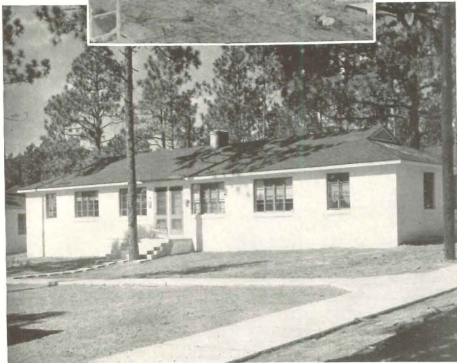
Entrance detail, and typical two-apartment block
