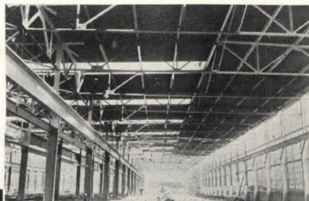
• Above: Milcor Steel Roof Deck being applied on new plant of A. O. Smith, Corp., Milwaukee, Wis. • Below: 1140 squares of Milcor Roof Deck were required to cover the huge Smith plant constructed as part of the national armament program.
