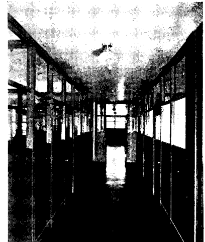
Office partitions are metal and glass
