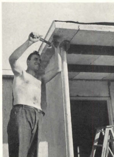
Built in an experimental housing project of the RSA at Alexandria, Va., these houses of precast concrete are now reaching completion, from plans by Kastner and Hibben, architects. Slabs are used for floors, walls and roof, with a board type insulation above the roof slabs. Houses of stabilized earth block and of rammed earth are also part of the project
