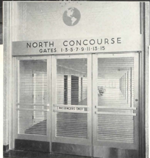
Above: All-glass doors of TUF-FLEX, made by Libbey-Owens-Ford, provide a full view of the passenger concourse.
