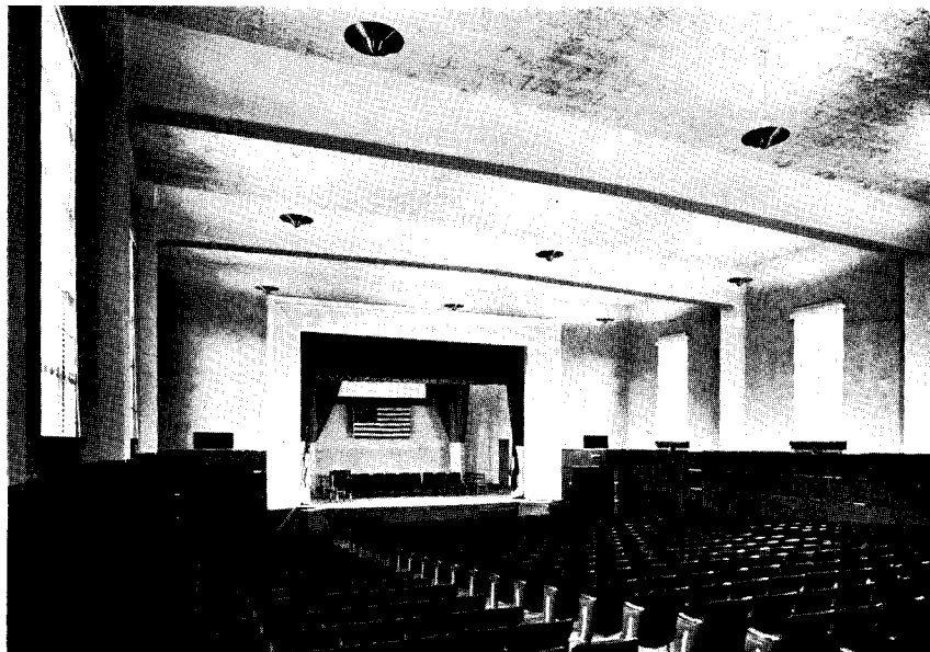
AUDITORIUM has exposed, rigid, concrete framing
