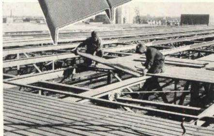
• Above: Milcor Steel Roof Deck being applied on new plant of A. O. Smith, Corp., Milwaukee, Wis. • Below: 1140 squares of Milcor Roof Deck were required to cover the huge Smith plant constructed as part of the national armament program.
