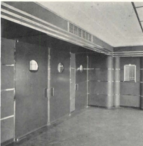
AUDITORIUM ENTRANCE: will intensive use justify such areas as this in the school of the future?
