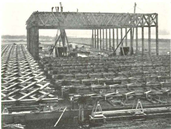
Trusses hoisted into place from trestles on which they were assembled; below, exterior views show assembly portion
