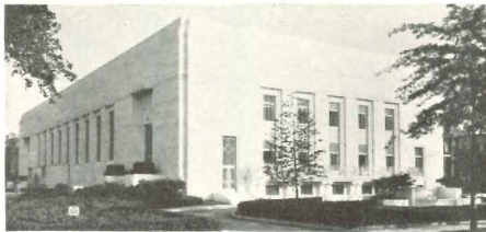
Above, Department of Commerce Bldg., Washington, D. C. Equipped with HOLTZER-CABOT Fire Alarm, Watchmen's Patrol, and Other Signaling Systems.
