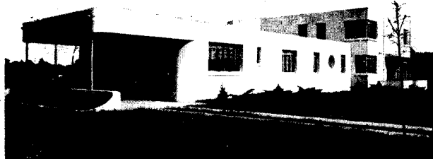
City Hospital, Cleveland, Miss. Overstreet & Town, Architects. G. C. Gardner, Builder.
