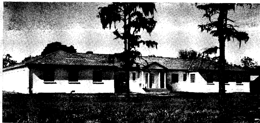
Lake Shore Hospital, Lake City, Fla. Ray Littlefield, Architect. Built by WPA. Cost (1940) : $40,000
