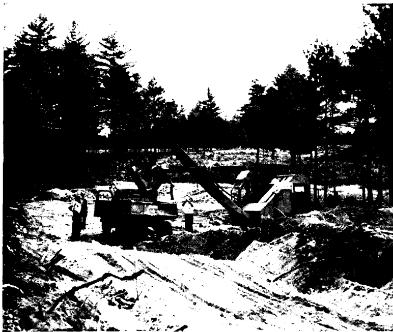
MARCH, 1940: Work on new site under way
