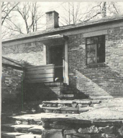
FRONT DOOR (Garage at left)
