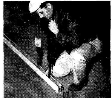
NO PREFABRICATED UNITS NECESSARY. The exclusive new metal base of the Gold Bond 2" Solid Partition System can be quickly cut and bent on the job. Plastering goes faster—and the finished job is more satisfactory.
