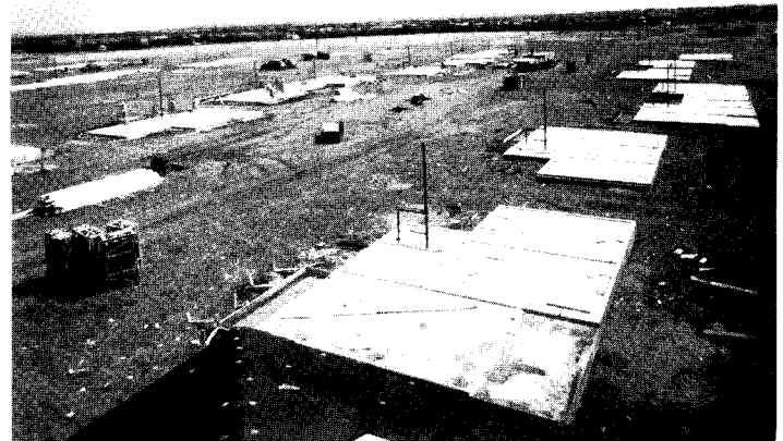
CONCRETE SLAB FLOORS and foundations
