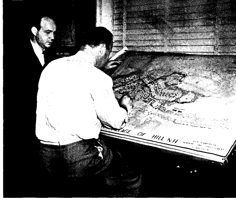
NOVEMBER, 1939: New site selected, design well under way
