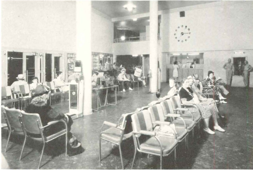
MAIN WAITING ROOM
