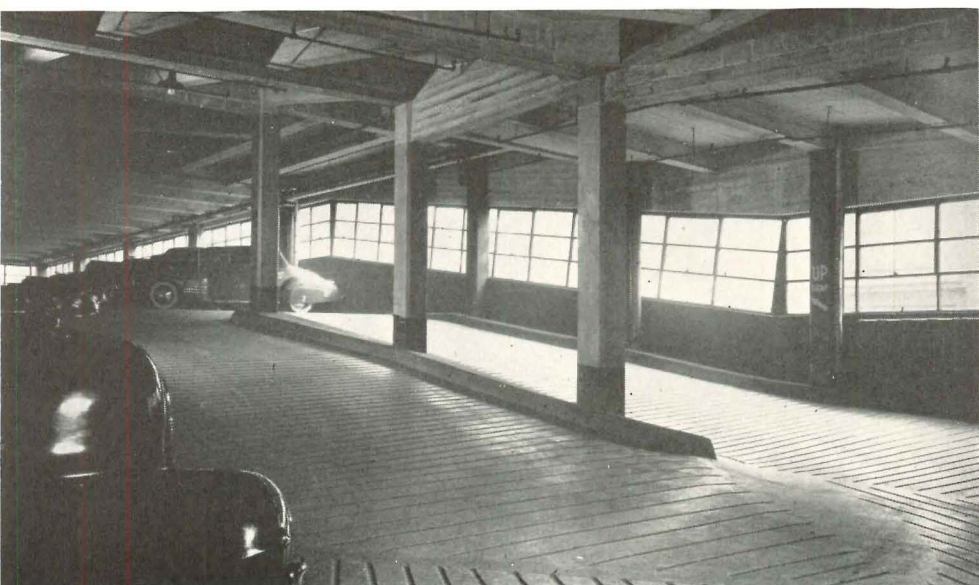
PSF PARKING GARAGE, PHILADELPHIA, PA.; HOWE and LESCAZE, ARCHITECTS. This garage, with shops on the first floor, almost achieves the “open” construction suggested above.
