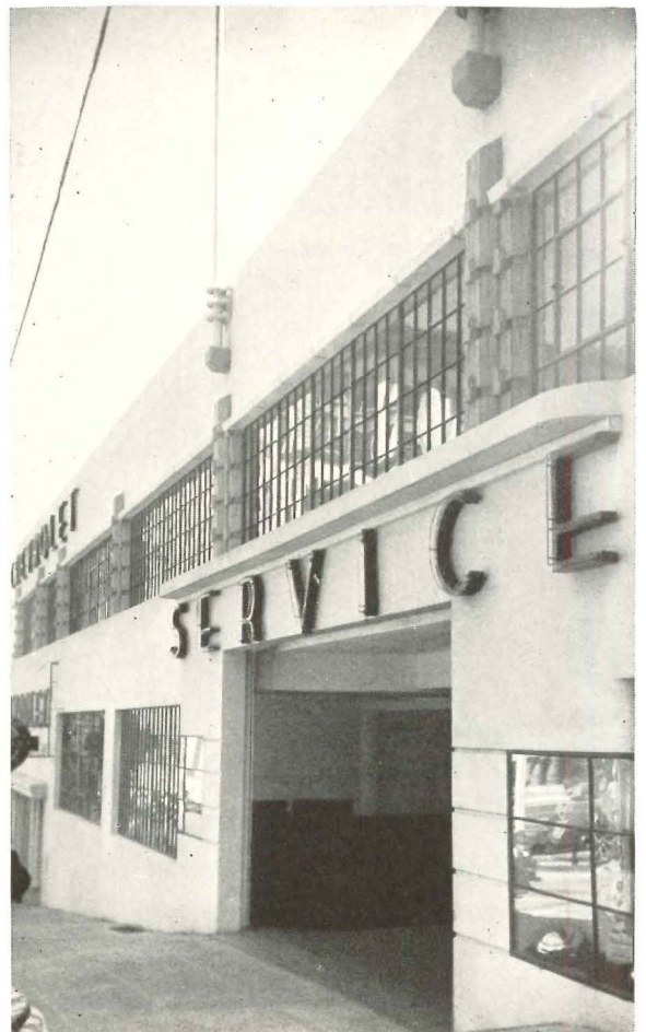
INGOLD CHEVROLET SALES AND SERVICE, SAN FRANCISCO, CALIF.; JOHN EKIN DINWIDDIE, ARCHITECT. This project has a downtown, sloping site, so service department is entered from upper level on side street, lower floor gains display space on a main street. Third floor houses heavy repairs, etc. Customer space on second floor has window overlooking new car salesroom. Construction is concrete, with widely spaced columns to allow easy manoeuvring.
