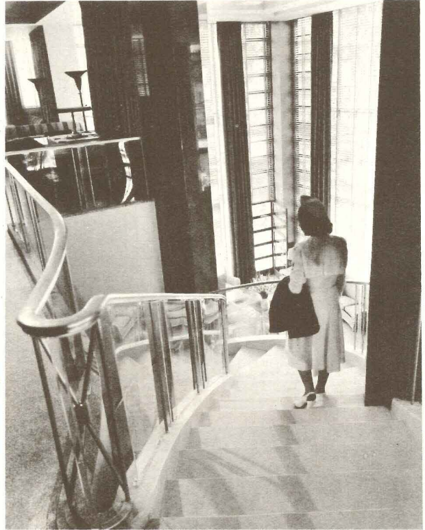
FREESTANDING STAIRS TO MEZZANINE have an etched clear plastic balustrade and aluminum handrail
