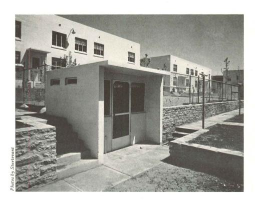
THE BUILDINGS at Holly Courts have concrete foundations, walls, floor slabs, and stairs. Roofs are of composition laid over wood trussed rafters. Interior partitions consist of 2-in. solid plaster on metal lath and steel studding; between apartments, partitions are sound-proofed. Steel casements are used throughout. Heating is accomplished by individual unit gas heaters. Floors in kitchens and baths are of linoleum;
