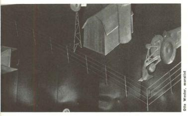
TEEL Steel in various forms and finishes is widely used for decorative puroses at the New York Fair. Here objects in low relief are mounted on a ackground of sheet-steel panels . . . Because of steel's strength and ductility, etails such as the fence can be easily executed in three dimensions.
