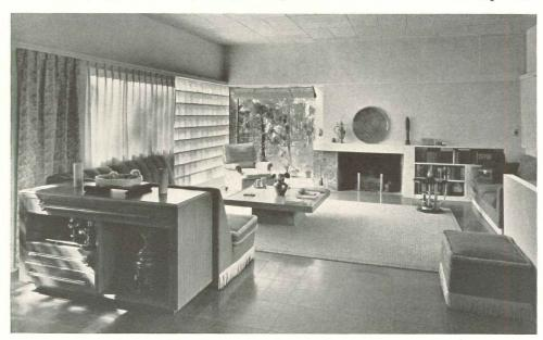
Glass block and plate glass in alternate panels vary the light transmission for living area
