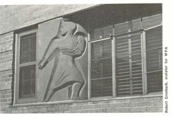
PRECAST CONCRETE spandrels were an organic part of the design of this USHA project in Buffalo. Designs were specially made for easy mass production on site.
