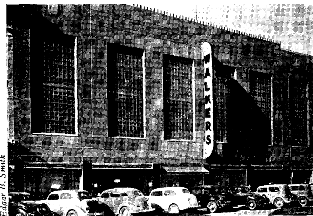
Fig. 21. The new exterior of Walker Department Store, Wichita, Kan., is of 1 3/4-in. precast slabs, up to 4 by 6 in. in size, faced with dark green crushed marble exposed by brushing. Lorentz Schmidt, Architect. At left, exterior before remodeling.
