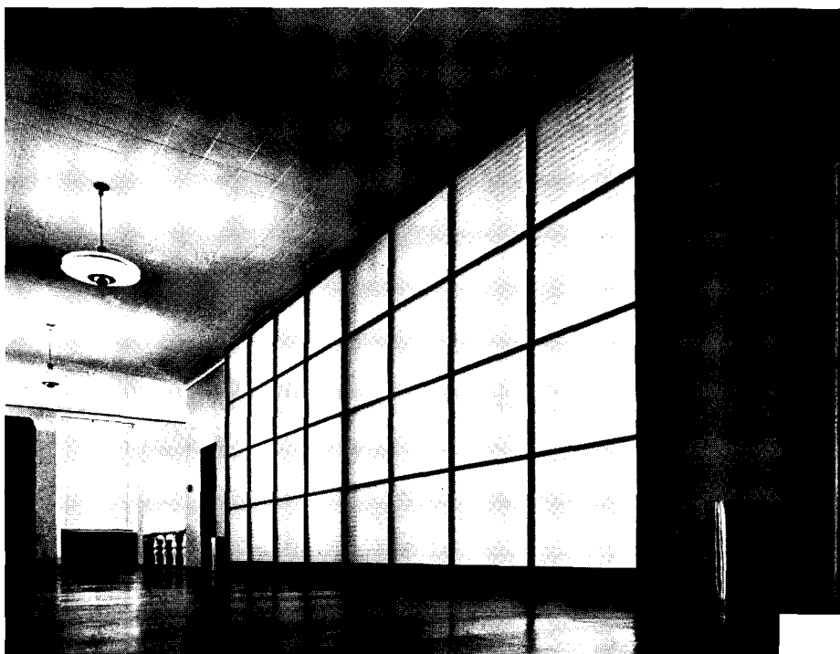
Business office of the first floor. Translucent-glass panels provide maximum light, as well as flexibility for possible changes in plan.
