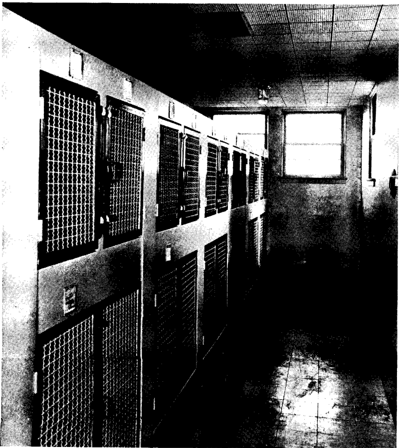
Kennels for sick animals: A cane-fiber material (Acousti-Celotex) applied to the ceiling deadens the din of barking.
