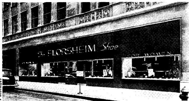
Fig. 22. Highly polished slabs, 2 in. thick, made with a mixture of blue and green granite chips, were used in remodeling this store in New York City.
