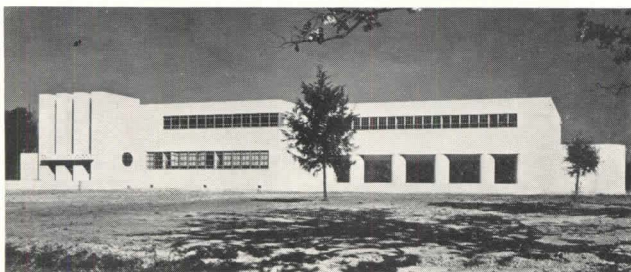
Fig. 12. Notable success in the use of concrete in the Columbia, Miss., high school. N. W. Overstreet and A. H. Town, Architects.
