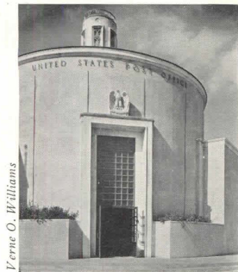
Fig. 11. Concrete walls, formed against plywood, were used in the Miami Beach, Fla., post office. Howard Lovewell Cheney, Consulting Architect for Procurement Division, Treasury Department.
