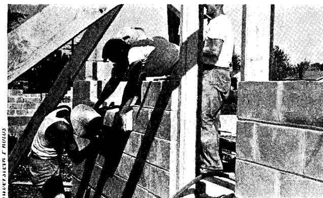
Fig. 25. Interior and exterior faces of hollow double concrete-masonry walls are usually finished with a portland cement paint.
