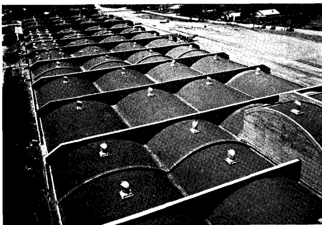
Fig. 7. Longitudinal barrel shells make up the roof of the Armstrong Tire and Rubber Co. factory, Natchez, Miss. Within the building, bays are 40 ft. wide and columns are 50 ft. apart in the longitudinal direction. J. T. Canizaro, Architect; Roberts and Schaefer Co., Engineers.
