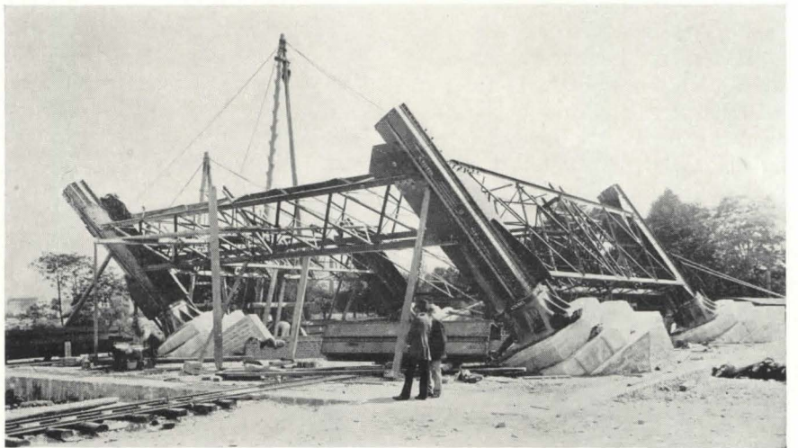
Fig. 6. Although worked in wrought iron, Eiffel's detailing of structural members would be quite adaptable to modern riveted steel construction. Photo taken July 18, 1887.
