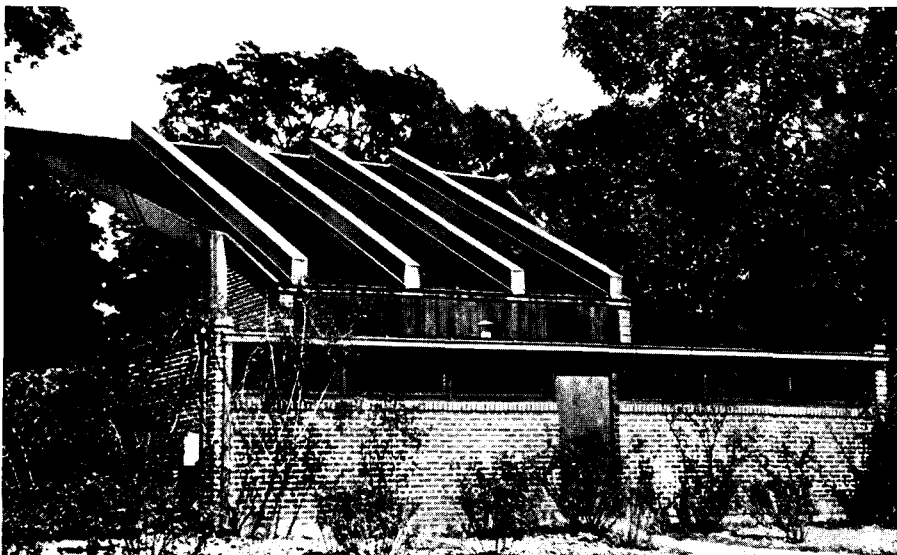
A tool shed and toilets for men and women are part of the design problem.
