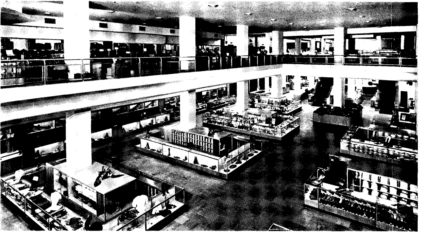
Main floor, new building. Column rows are aligned; but in the new structure every other row has been eliminated.
