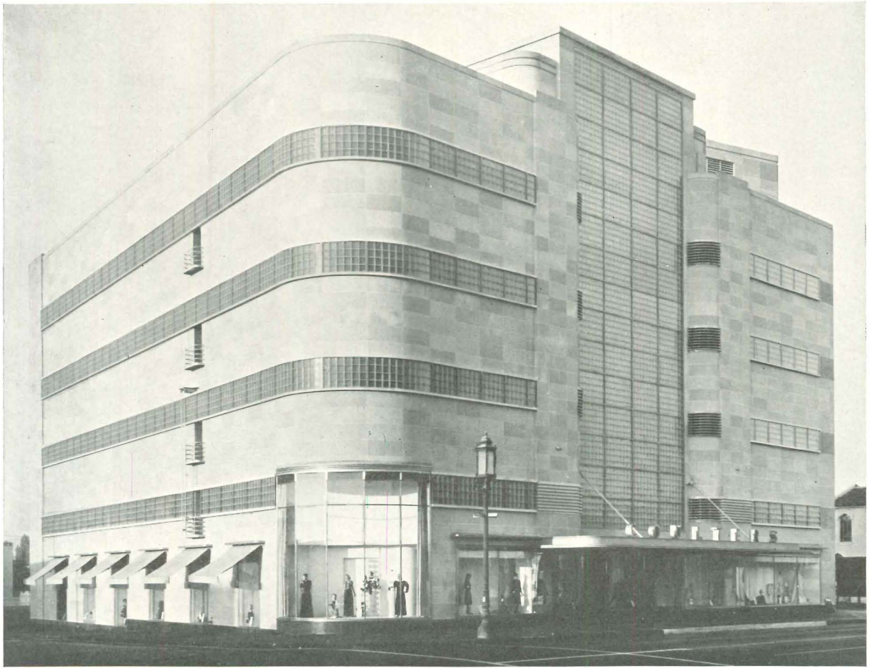
Coulter Department Store, Los Angeles. Reinforced-concrete walls are "blocked" to simulate Bedford limestone; several brands of Portland cement are used in the brush coat to give the different color tones.
