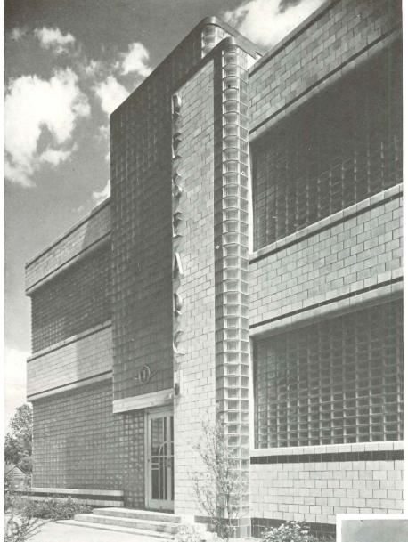
BUILT to house the technicians engaged in the development of glass products, this office building is essentially an airtight, well insulated enclosure. Various patterns of glass block were determined by the orientation of the building: a higher percentage of light transmission was allowed on the east and north where solar radiation is low; but on the west and south, blocks were specified to reduce solar radiation. Interior corridors are well lighted by means of full-height glass partitions.
