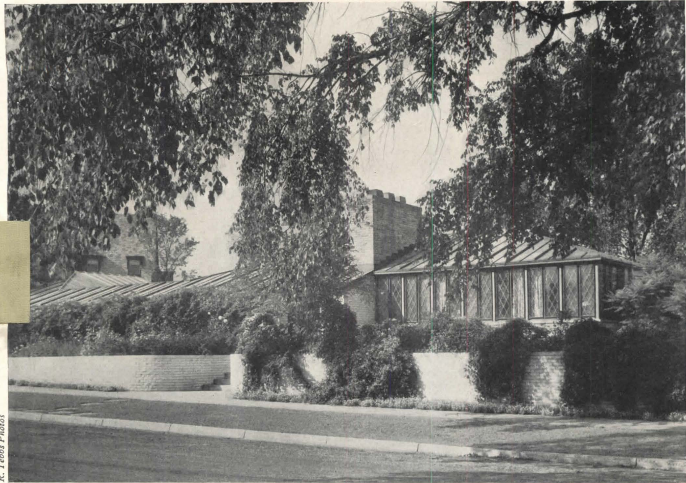
General view, conservatory roof at extreme left
