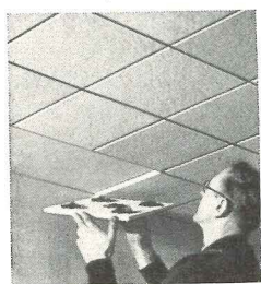
Showing easy application of BLENDTEX Tile to ceilings, using adhesive.
