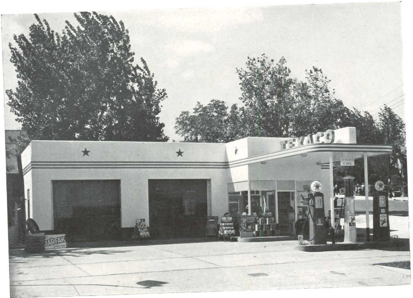
REMODELED "T" TYPE STATION at Wenatchee, Washington. Sheet metal facing throughout.
