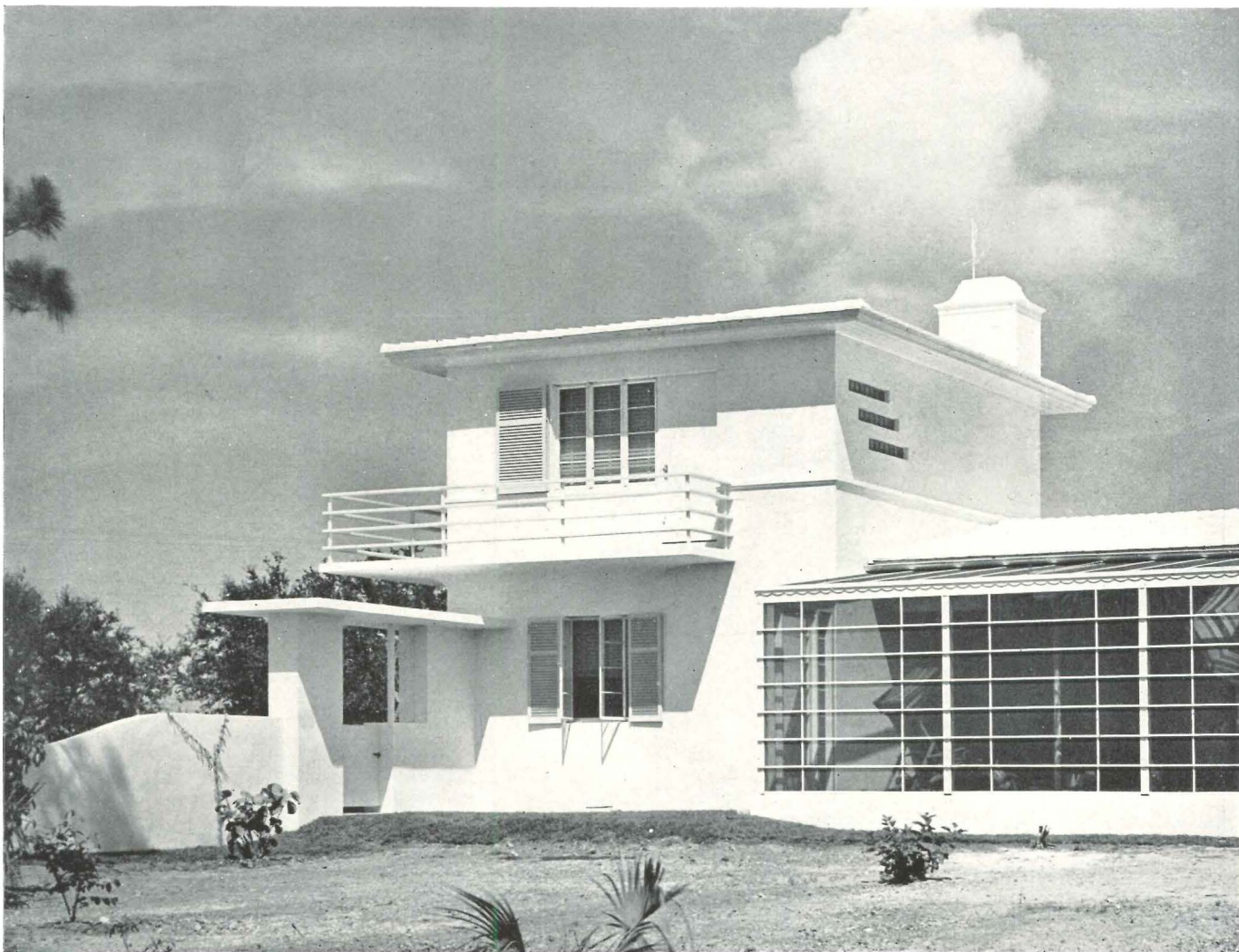
VIEW SHOWING PATIO SCREEN
