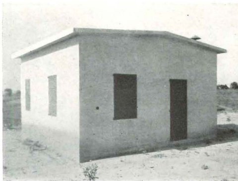
SOME OF PUERTO RICO'S MANY STRAW HUTS HAVE BEEN REPLACED by these modern hurricane-proof houses. Monolithic in construction, designed to resist horizontal wind velocities up to 150 m.p.h., they have flat or nearly flat concrete roofs not subject to wind pressure.
