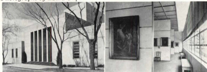
Taylor Museum, Colorado Springs, John Gaw Meem, architect (1935). Showing unit system for removable display partitions
