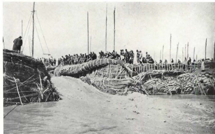
WHERE MODERN MACHINES COST MORE THAN COOLIE LABOR men push and roll the willow "sausage" to its final resting place as their ancestors did thousands of years ago. As the gap is narrowed, the rush of the water is greater, but the "sausages" are firmly fixed by rope and sticks.
