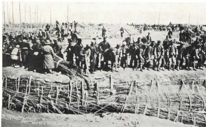
IT TAKES ONE HUNDRED MEN to roll the "sausage" to the gap. When the fascines are set in place one above the other, they are spiked and tied together with rope, and then covered over with earth and rocks.
