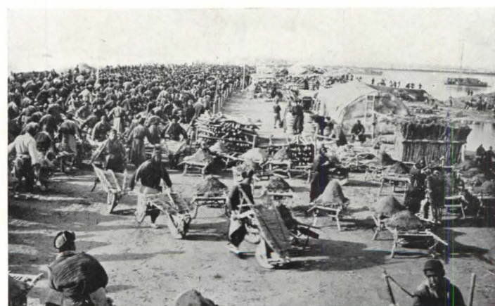
WHEELBARROWS WOVEN FROM WILLOW BRANCHES and manned by coolies, carried supplies to danger points on levees. Wheels and framework are hand hewn, and fastened with hemp rope.
