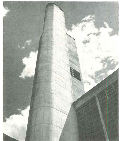
2 3 1 Interior view of the machine hall; at the far end is the mezzanine where the control room is located. 2 View of the stack, the cooling tower, the power-house and the machine laboratories. 3 The stack, showing the repetition of standard concrete forms.
