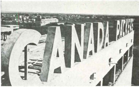
1 The free-standing reinforced concrete sign.
