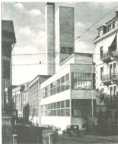
2 3 1 Interior view of the machine hall; at the far end is the mezzanine where the control room is located. 2 View of the stack, the cooling tower, the power-house and the machine laboratories. 3 The stack, showing the repetition of standard concrete forms.
