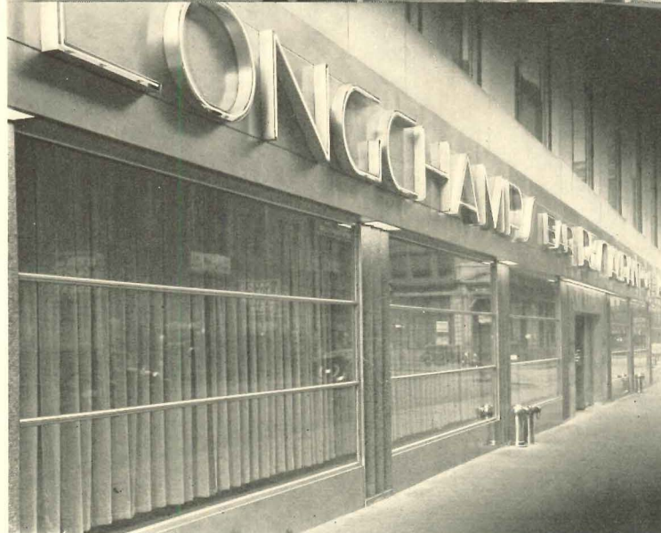
Exterior, Longchamps Broadway Restaurant, New York City. Broad horizontal windows and metal lettering containing neon tubes produce effective exterior treatment.
