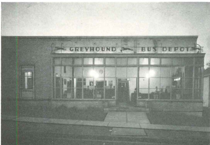
BUS TERMINAL FOR THE ATLANTIC GREYHOUND LINES, MARTINSVILLE, VIRGINIA—GEORGE D. BROWN, ARCHITECT
