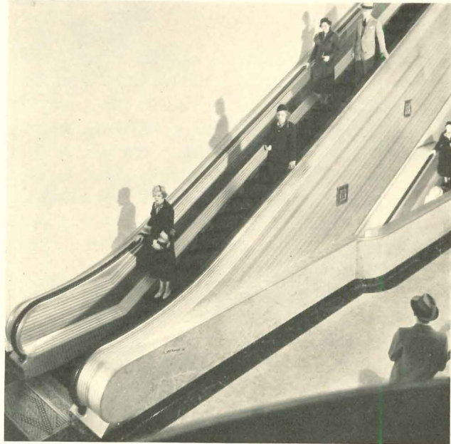
ESCALATOR, MARSHALL FIELD & COMPANY STORE, CHICAGO, ILL. GRAHAM, ANDERSON, PROBST & WHITE, ARCHITECTS. To derive greatest benefit, escalator should be centrally located.
