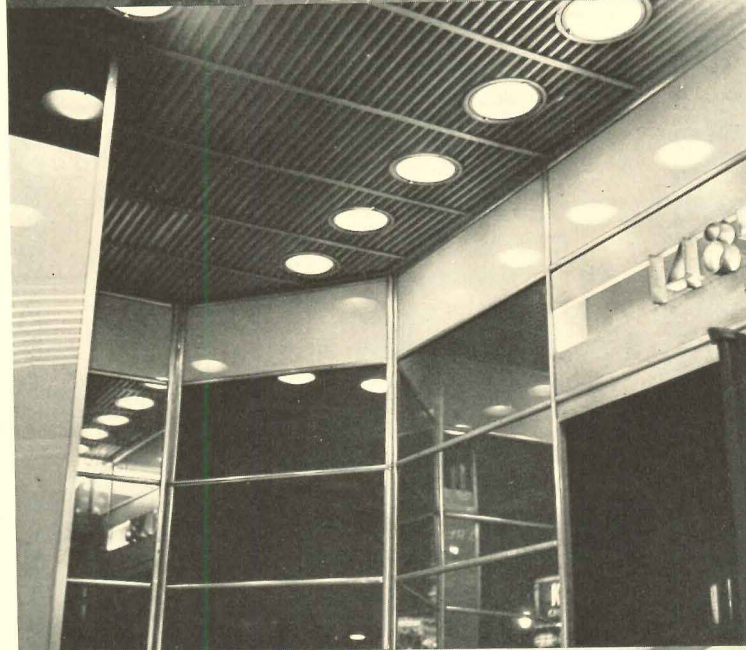
Detail of entrance, Childs Restaurant, New York City. Use of colored mirrors and glass in metal frames.
