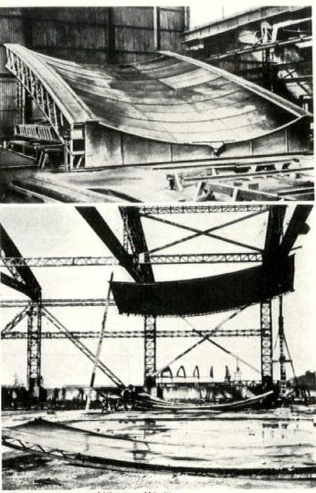
standardized roof sections are fabricated in advance and then quickly assembled on the site
