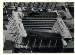
The shopping center throws tradition overboard. In plan and elevation a spiral, its courtyard profile steps back for increased light; buttresses carry the corresponding overhang outside.
