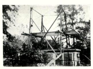
Another pioneer scheme by Robert C. Lafferty consisted of separate precast slabs for walls and floors erected in place on the site. Fourteen years ago adequate mobile cranes were not available, and a gallows frame with chain blocks had to be erected for the placing of the 3-ton slabs. Such slabs can now be easily placed with the new 8-ton automobile cranes. Where in 1922 it took 4 days to assemble a house, only 4 hours would now be required.
