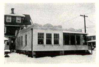
This dwelling was erected under the New York City Building Code in 1922. It consists of two structural units of the kind shown in the strength test photograph. The units were manufactured complete in the plant and transported more than 30 miles to the site.
