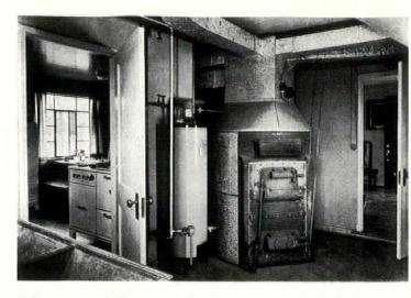
Utility room with heater and laundry is on ground level. The cement floor is supported on steel bar joists.
