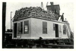
Back in 1922 completely prefabricated concrete structures—measuring 12'-6'' by 28'-6'' in plan and including floor and roof as well as walls—were produced from designs by Robert C. Lafferty, architect. The photograph shows a strength test of 31,000 pounds on one of these early prefabricated house units.
