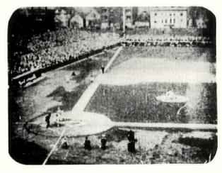
INCREASING PRECISION: Clearness in the television images depends largely on the number of scanning lines. The accompanying views are not photographs of actual television images, but photographic equivalents made by RCA to facilitate the study of images. Pictures now consist of 343 lines. An increase to 441 lines is anticipated.
