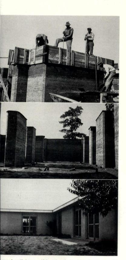
cammed earth houses — high cost ratio for labor, low for materials
