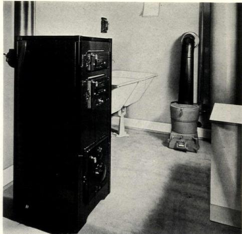
specially designed boiler for a hotater radiator heating system for provion of central heating; can be installed a one-floor home without basement. All equipment shown on this page prouced by American Radiator & Standard anitary Corp.)
