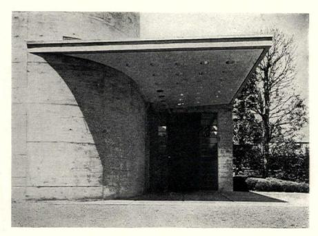
This concrete porte-cochère at the main entrance is cantilevered from two sides, meeting diagonally and resulting in a light construction. The under side is painted a light yellow.
