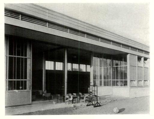
Each classroom faces east and west, opens through a wide door into an outdoor classroom into which the pupils' activities can be extended. Inclosed corridors are eliminated. The kindergarten faces south and opens into the attached play patio. Roof overhangs, supplemented by vertical awnings, eliminate much of direct sun radiation, but permit an abundant influx of light.
