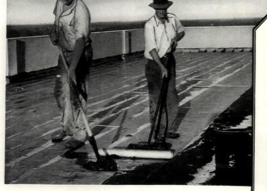
Thin copper in long sheets, 30" wide, combined with alternate layers of asphalt...ushers in a new phase of built-up roofing practice.
