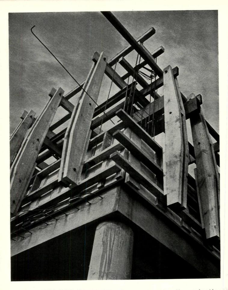
CONCRETE HOUSES UNDER CONSTRUCTION AT GENESTA ROAD, PLUMSTEAD, ENGLAND The concrete walls are fabricated by means of wood forms which extend a full story in height and can be used repetitively for successive pourings of concrete as the building goes up from the foundations.
