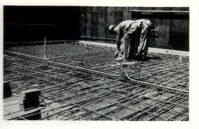
ABOVE: Notice the generous use of heavy steel reinforcing rods in the floor slab. Ribbed concrete walls were reinforced equally well. RIGHT: This photograph shows how the new "flexible" steel forms are fitted to one another. They come in sections and are fitted together by means of screws to the other side sections, thus making it possible to build walls of any thickness required. BELOW: Pouring concrete into flexible steel forms.
