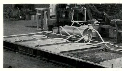
tests at Yale show that vacuumizing speeds up hardening of concrete columns and floors
