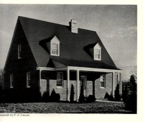
This house indicates the possibility of home construction under the FHA. The house is of brick-veneer construction, with unfinished attic space convertible into two extra bedrooms and bath. A sales price of \$5,500 includes improved lot and all mechanical equipment—furnace, hot water heater, electric range and refrigerator, sewage disposal system, drilled well with electric pump. Contractor's allowance and sales-promotional expense are included in sales price.
