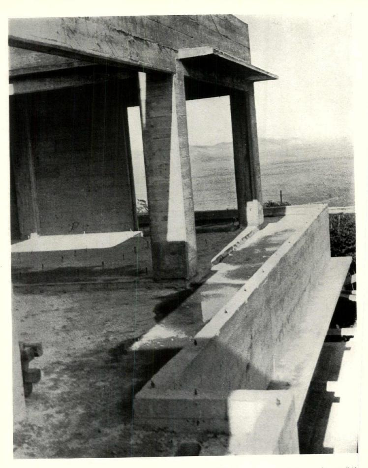
A COUNTRY HOUSE OF CONCRETE IN JAPAN ANTONIN RAYMOND, ARCHITECT Formwork has just been removed, showing the monolithic construction. Roofs, columns and walls, window overhangs and floors, all are cast together without joints. Floor bolts, downspouts, piping and ducts are set in the forms before the concrete is poured.
