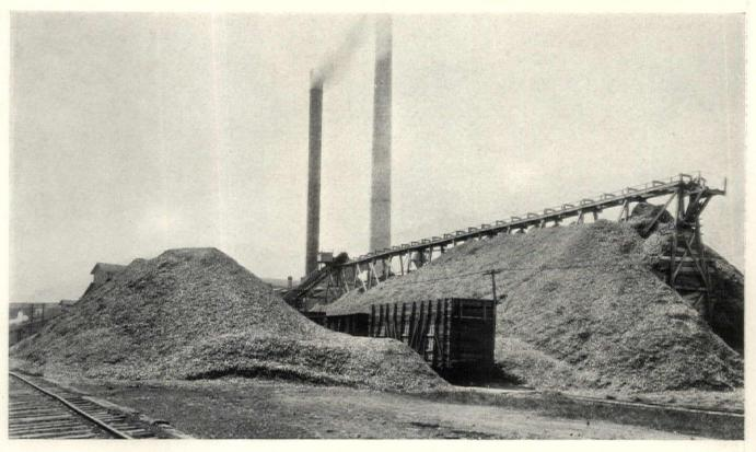
Stocks of waste wood and wood chips, ready for fabrication into insulating materials, at plant of Wood Conversion Company, Cloquet, Minnesota.
