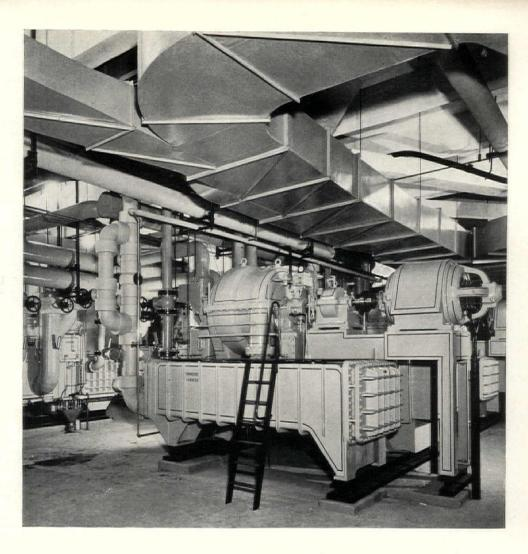
Centrifugal-type refrigeration machines using a nontoxic refrigerant in conjunction with air conditioning.
