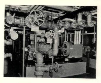
(Left) Elevator machines for handling passenger cars traveling at the rate of 1,400 feet a minute. (Right) Electric-driven fire pump for maintaining an adequate water supply for fire standpipes.
