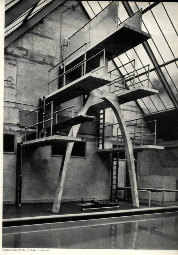
REINFORCED CONCRETE DIVING STAGE AT END OF SWIMMING POOL
