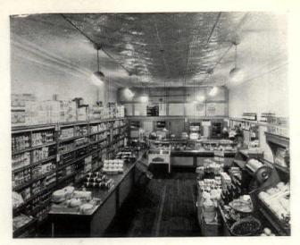
LIGHTING OF A TYPICAL COUNTRY CHAIN FOOD STORE. IN THIS CASE THE EQUIPMENT FOLLOWS TRADITION, IN IN THAT IT IS SUSPENDED FROM THE CEILING, BUT IT IS SIMPLIFIED IN FORM AND LIGHT IS EMITTED ONLY IN THE DIRECTION OF THE MERCHANDISE.
