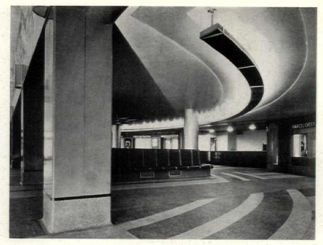
General view of concourse in the new railway station at Hamilton, Ontario, in Canada. The wainscot, doors and frames, counter grilles, column coverings and walls are all steel. The walls are finished in baked enamel of a deep terra cotta color. The column coverings are also of steel, finished in bright aluminum enamel.
