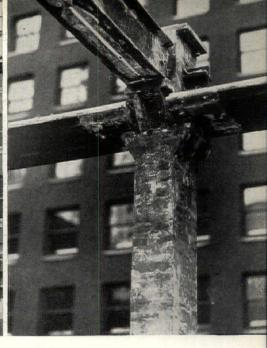
(Left) This picture, taken from the street, shows stripped column near third floor level. (Center) Masonry removed from exterior columns demonstrates that the walls were supported by columns. (Right) Head of a column at the fifth floor level.
