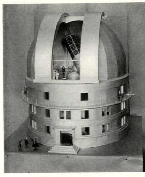
(Above) Model of McDonald Observatory for University of Texas showing great reflecting telescope with its 80-inch mirror and 62-foot revolving dome. When erected on Mt. Locke, it will be the second largest in the world. Length of tube—2 feet. Total weight of moving parts of telescope—45 tons.
