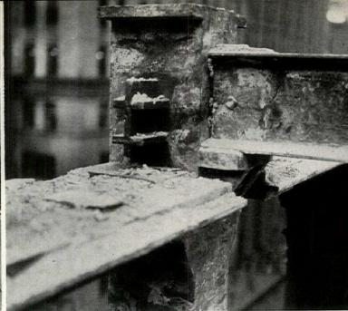
(Left) Committee examining exposed column of the fifth floor of the Home Insurance Building. (Right) Close-up of head of column at fifth floor level, LaSalle Street front, showing wrought-iron floor girders and cast-iron lintel in place with the spandrel I-beams removed.
