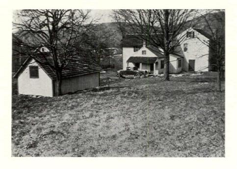
The wing of the old house (illustrated a left) was much too narrow for its heigh Its overhanging roof was eliminated, th tall narrow chimney rebuilt to accommo date three fireplaces, and the fenestra tion changed, and a tool room and go rage added to improve the south eleva tion and to give the house a greate width.
