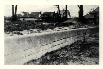
Figure 6. Water accumulated in this wall and froze, exerting forces that rival the power of dynamite. The effect of rapid wetting and slow drying.
