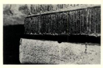
Figure 4. Dense cement mortar poorly adapted to dense impervious Water entering shrinkage cracks cannot subsequently evaporate through the dense solid materials.
