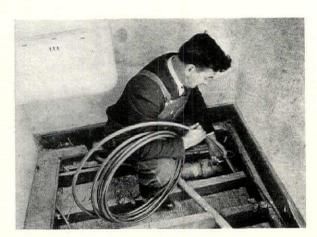
FLEXIBLE COPPER TUBING CAN BE READILY INSTALLED IN OLD PARTITIONS; NO FITTINGS REQUIRED; ECONOMICAL. DIAMETER UP TO 11/4": UP TO 60 FEET IN LENGTH: ORDINARILY SUPPLIED IN 20-FOOT LENGTHS.
