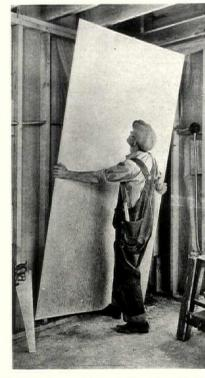
VIEW SHOWING APPLICATION OF LARGE SHEET OF PLY-WOOD OR INSULATION BOARD, WITH BOARDS REACHING FROM FLOOR TO CEILING, SMOOTH FLUSH SURFACES ARE OBTAINED WITH A MINIMUM OF JOINTS. COMMON WIDTH IS 4 FEET, LENGTHS FROM 8 TO 12 FEET.
