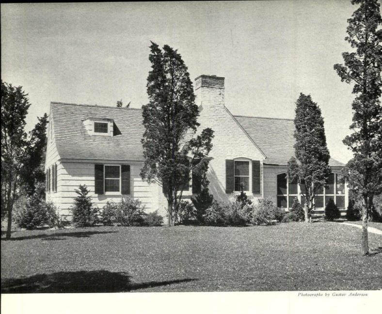
Construction: walls and roof of wood shingles. Oak floors. Steam heating. Color scheme: white walls and green roof. Cost (house completed in 1933): \$6,100.
