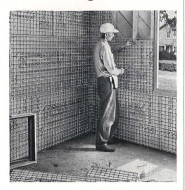
A plastering job is no better than its base. A good plastering job deserves a good base. Build for greater permanence by using Pittsburgh Steeltex Plaster Lath: It adds **strength** where **strength** is needed.
