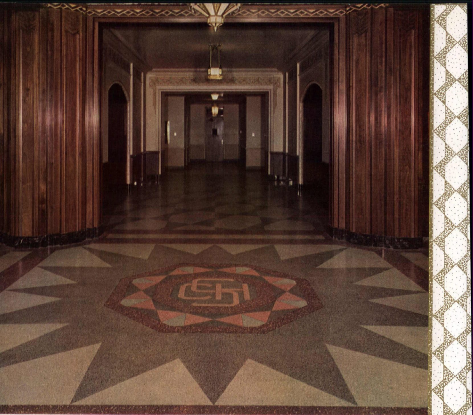
Terrazzo floor made with Atlas White portland cement in City Hospital, Springfield, Ohio. Letbly, Eastman & Budke, Springfield, architects. Tulsa Terrazzo & Mosaic Co., Tulsa, Okla., terrazzo contractor.
