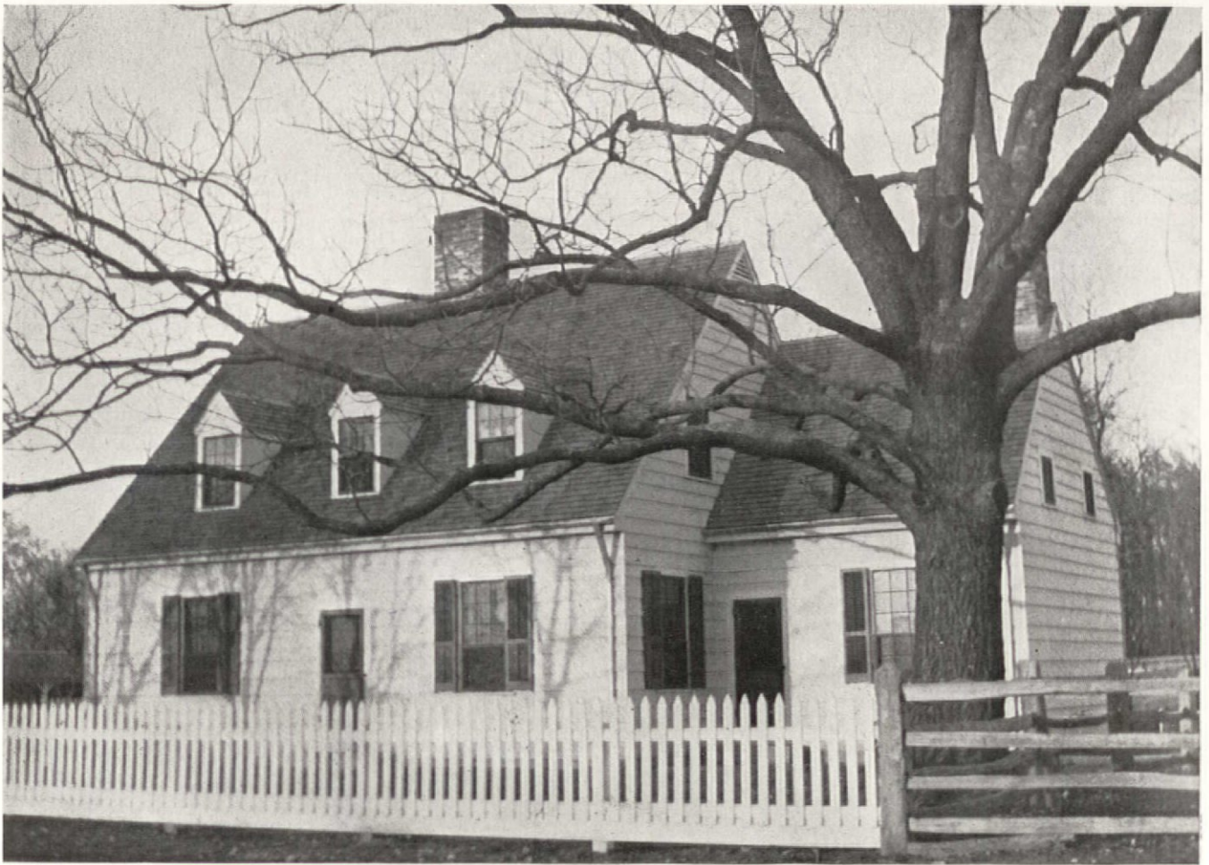
TENANT HOUSE ON ESTATE OF MRS. CAROLINE H. DUPONT IN KENT COUNTY, MARYLAND HENRY ATHERTON FROST AND ELEANOR RAYMOND, ARCHITECTS
