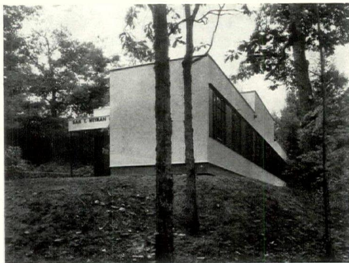
BIOLOGICAL LABORATORY OF HIGHLANDS, N. C., MUSEUM TUCKER AND HOWELL, ARCHITECTS OSCAR STONOROV, CONSULTANT
