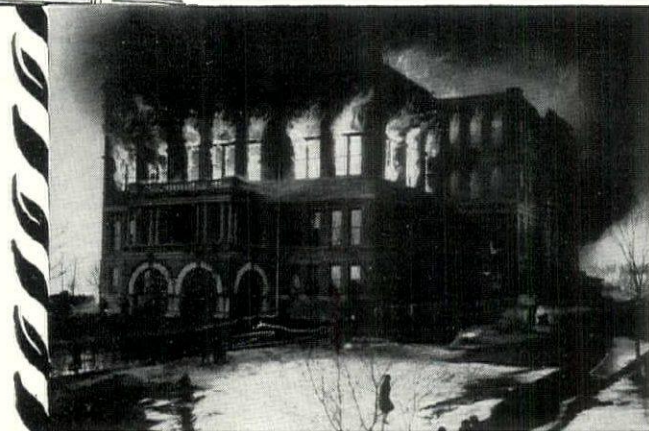
14 Diebold Vault Doors preserved priceless records in the destruction of the N. D. State Capitol fire Dec. 28, 1930.
