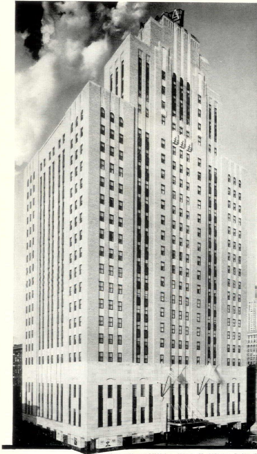
Lawson Memorial Y.M.C.A., Chicago, Ill. Architects—Perkins, Chatten & Hammond. General Contractors—Jacobson Bros.
