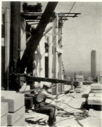
TOPPING OUT, BUILDING NO. 10
