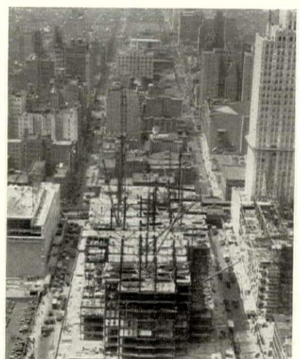
GENERAL VIEW MAY, 1932
