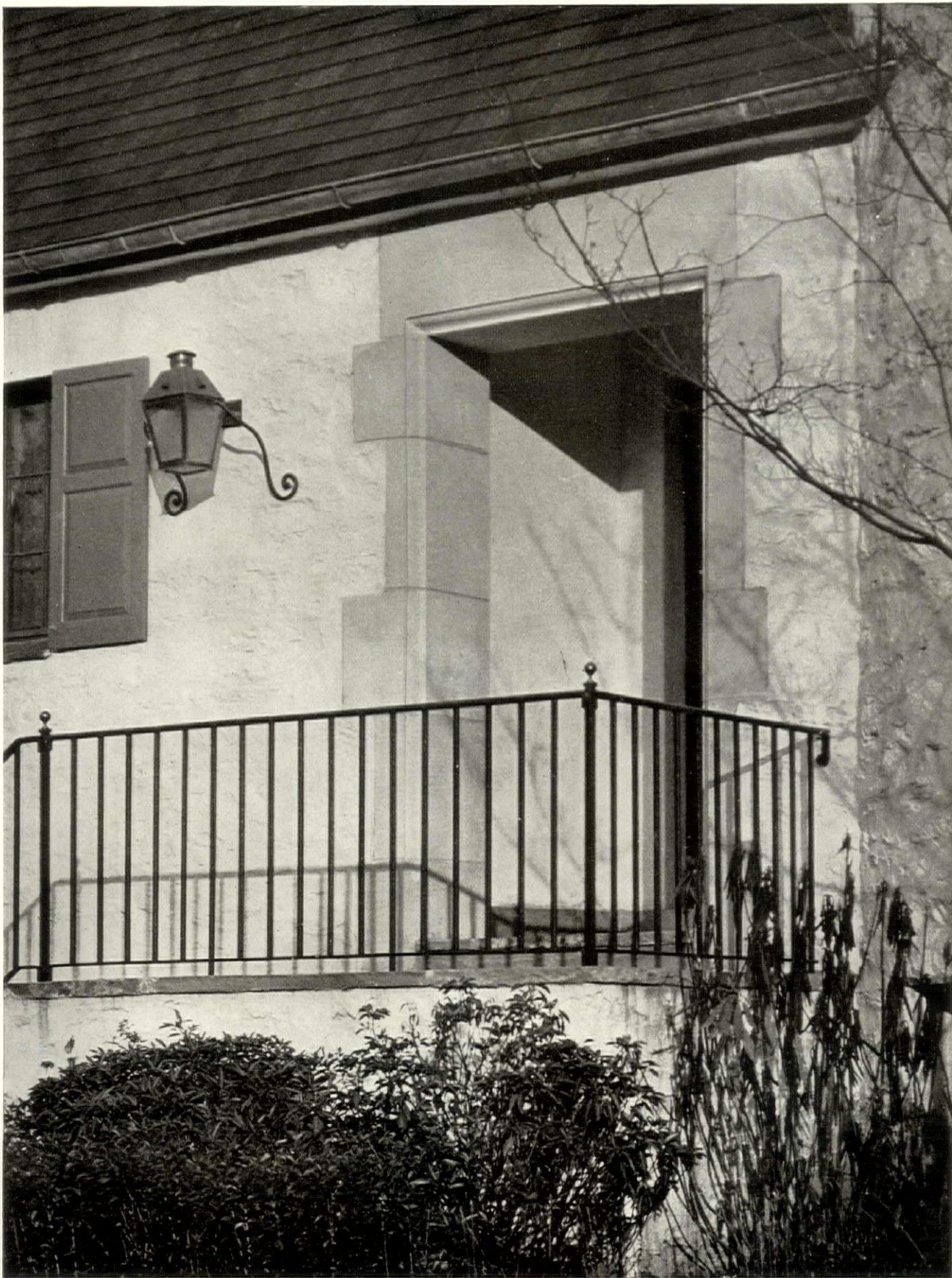
Detail of entrance.
